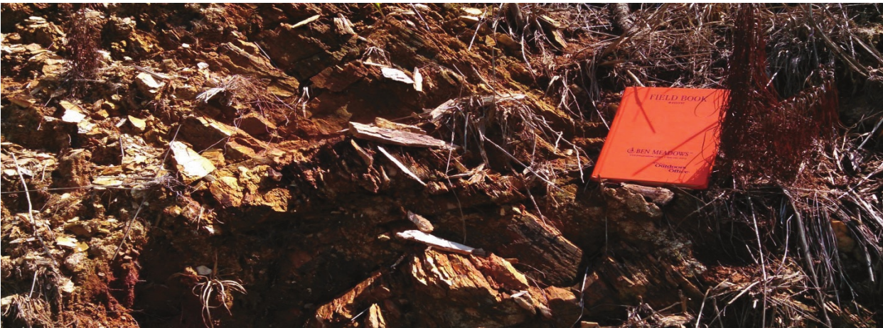
Photograph showing exposure of Quartzite Layer at Plant Wansley
