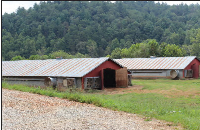
Four large chicken houses located at the confluence of Tuckaluge Creek and Warwoman Creek.
