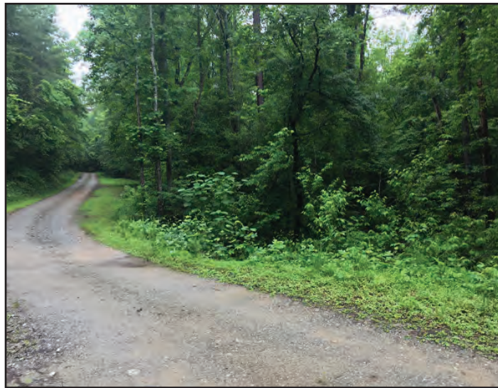
Gravel Forest Service roads throughout the Warwoman Creek watershed produce ongoing erosion and sedimentation into streams.
