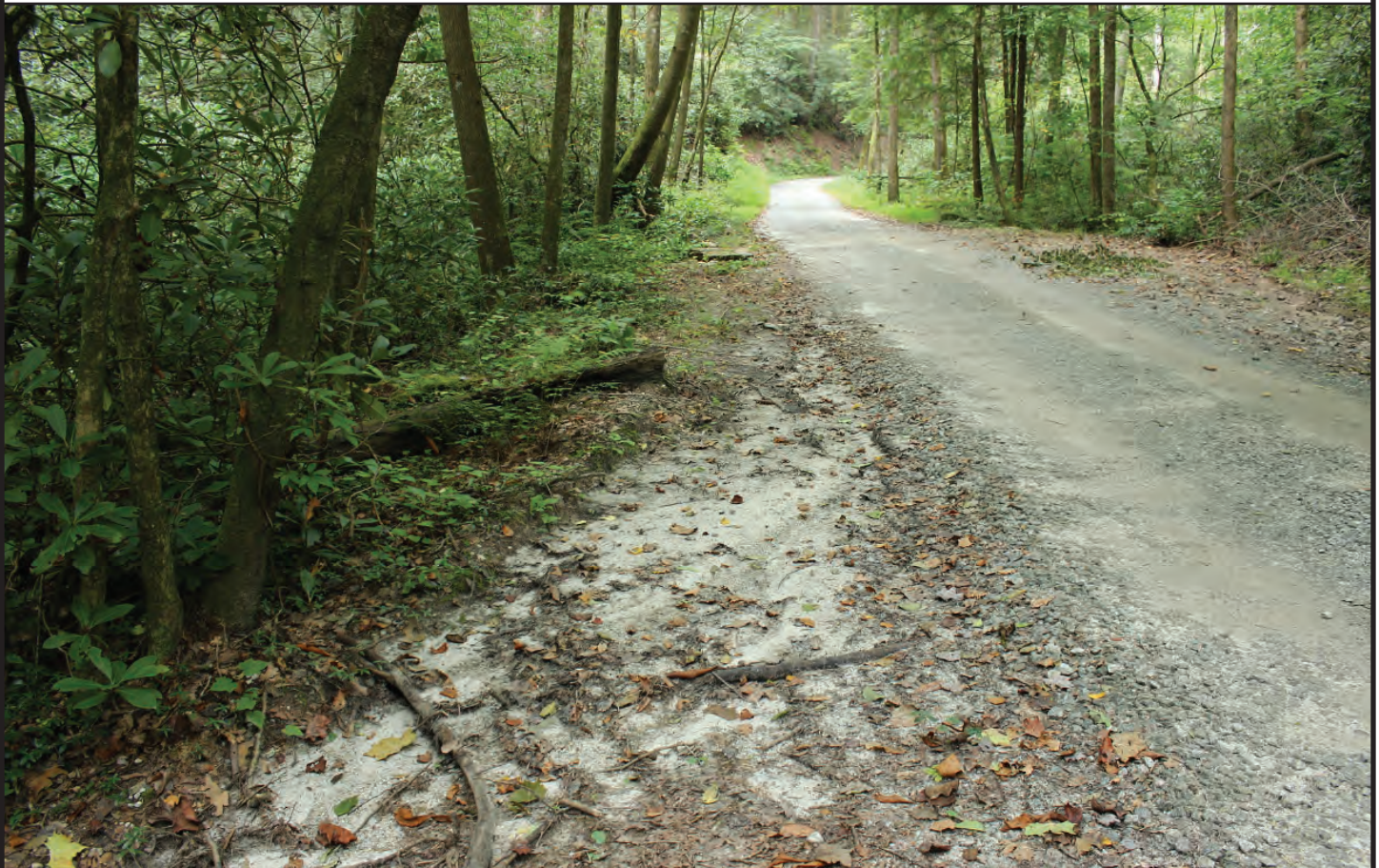
Sediment turnout from the gravel road through Warwoman Dell is directed toward Warwoman Creek. Even in the furthest upstream sections of the creek, sedimentation coming from unpaved roads is an apparent issue.
