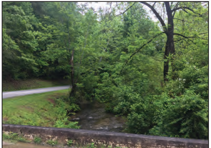
Warwoman Creek is crossed by a bridge on Sandy Ford Rd.
