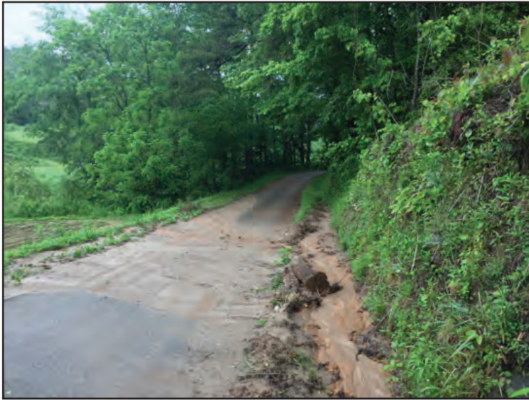
Sediment washes across a road near Big Creek. Without stormwater management, paved roads can contribute to increased runoff velocity and volume.
