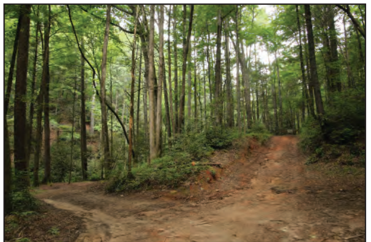
Runoff from FS 155A flows directly to Walnut Fork and one of its tributaries.
