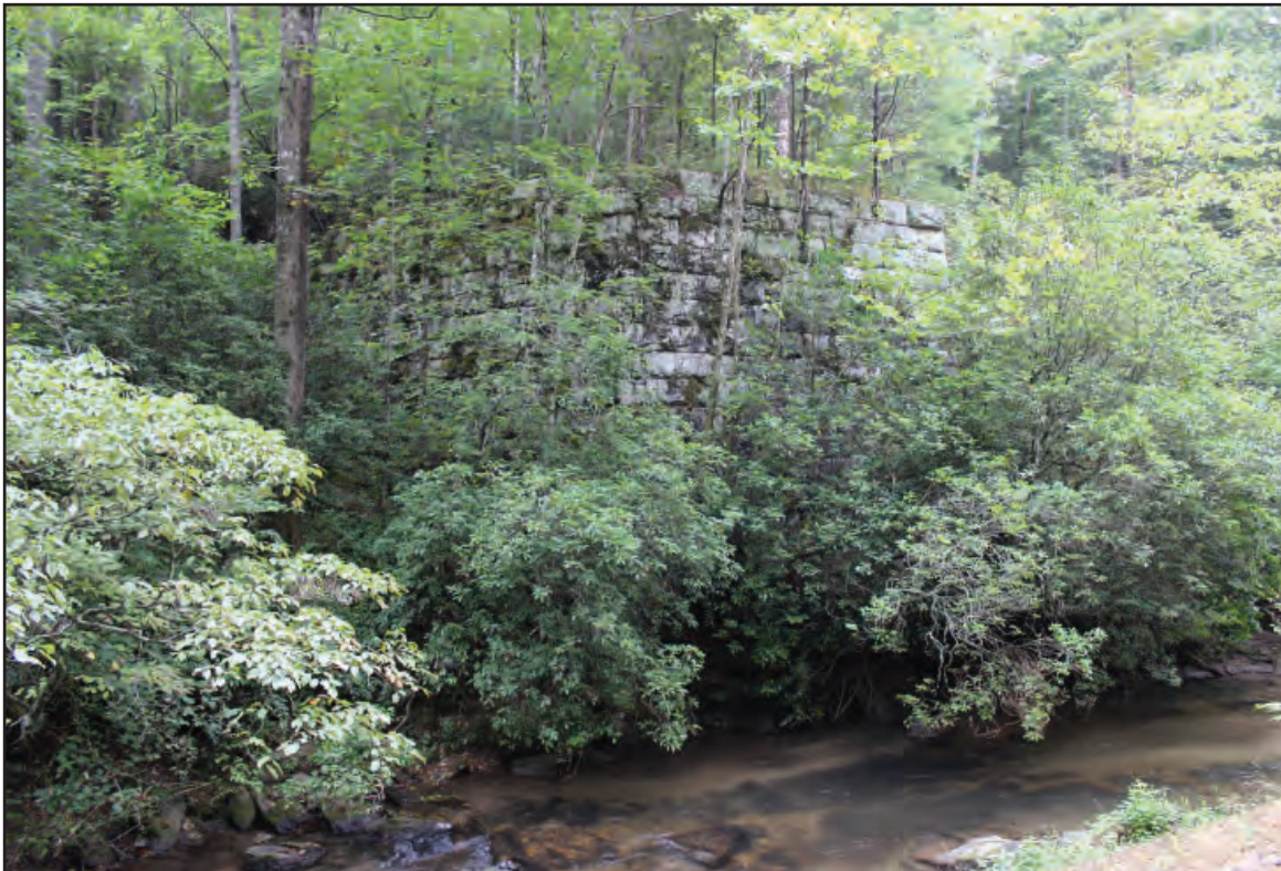
Remnants of an abandoned railroad truss alongside Warwoman Creek.
