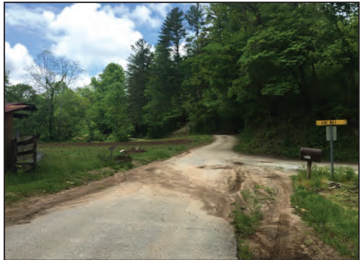
Sediment washes across and down Walking Stick Rd. toward Big Creek from farmland and dirt trails.
