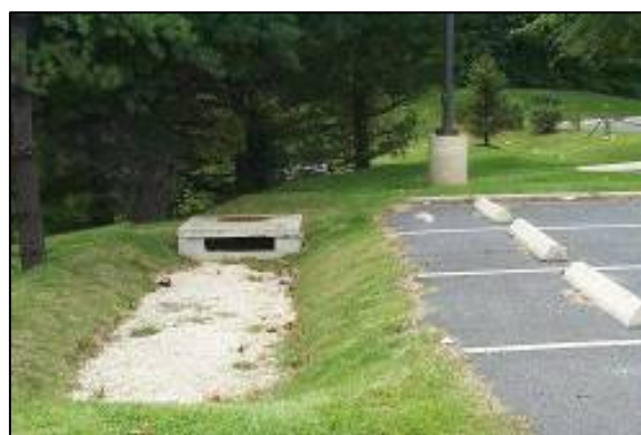
Figure 6.18: Infiltration Trench (Source: Center for Watershed Protection)
