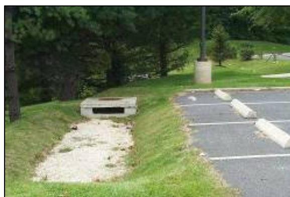
Figure 8.4: Infiltration Trench (Source: Center for Watershed Protection)
