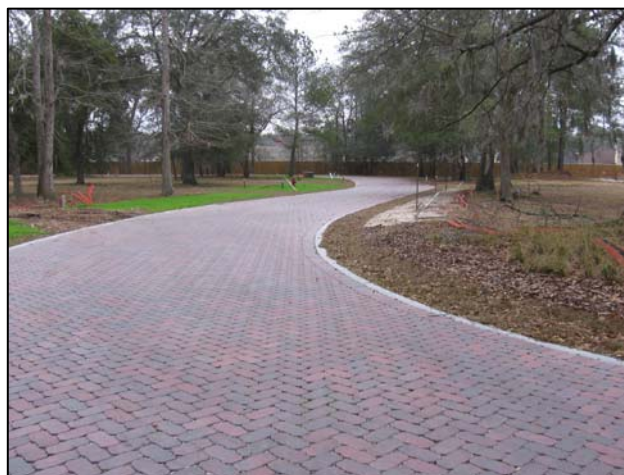
Figure 7.9: Reduced Street Width Used on a Residential Development Site
