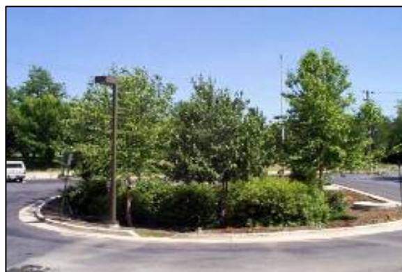
Figure 6.17: Bioretention Area (Source: Center for Watershed Protection)
