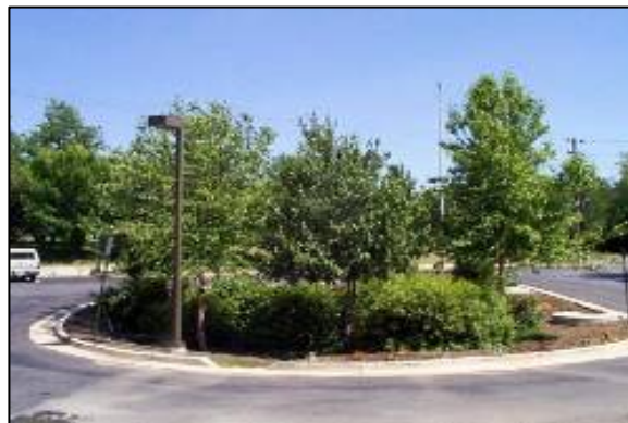
Figure 8.3: Bioretention Area (Source: Center for Watershed Protection)
