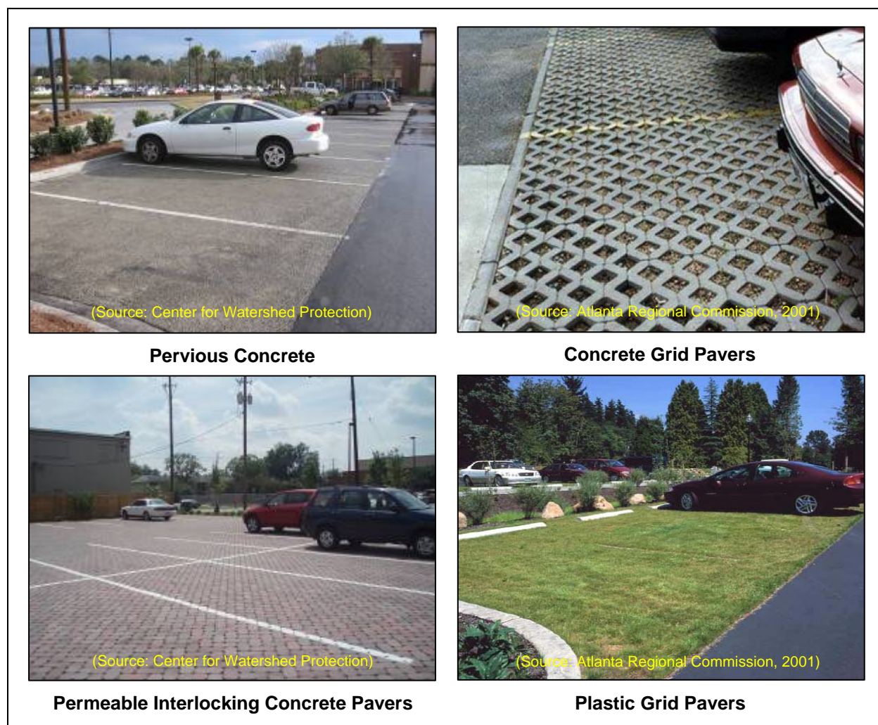
Figure 7.29: Various Permeable Pavement Surfaces
