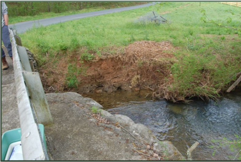
Figure 25. Eroding streambank at Buttrum Road Crossing.
