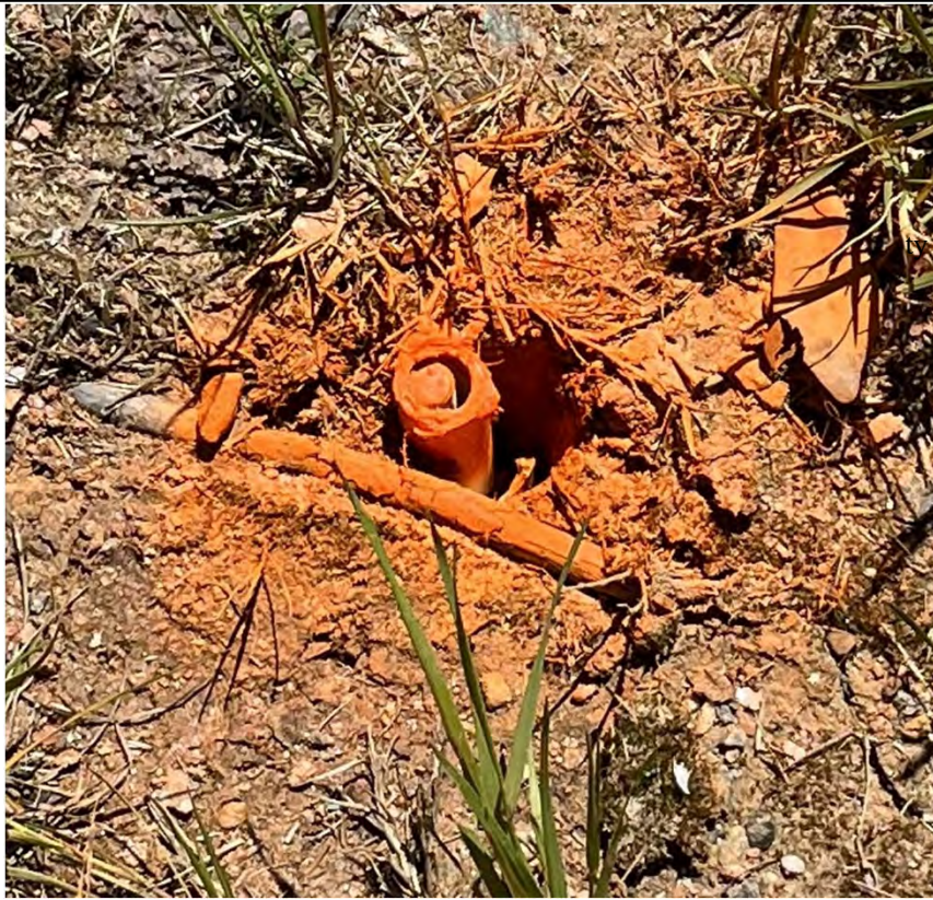
Photo 1 – Trench Marker (Typical Marker of 55, set at grade) – \frac{3}{4} " rebar set in 1-in PVC painted
