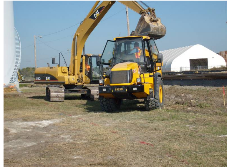
Photo 10: Excavation in area I.
