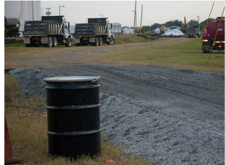
Photo 6: Dump trucks for soil removal
