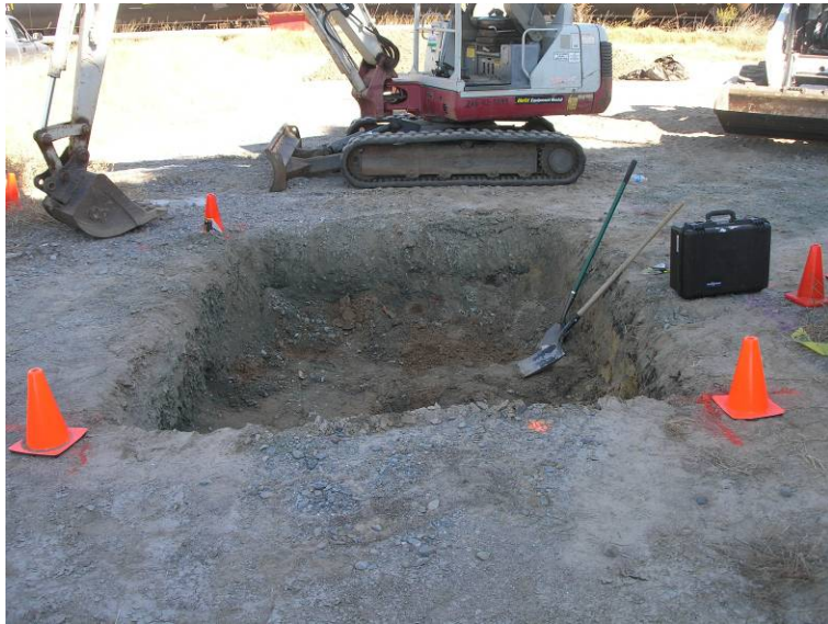
Photo 25: 2010 Area D Excavation
