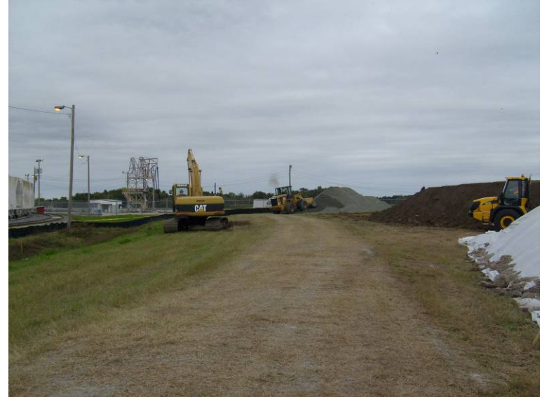
Photo 2: Site prior to excavation.
