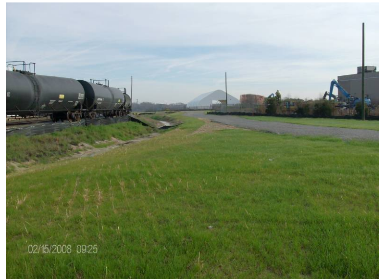
Photo 24: Restored excavation area.
