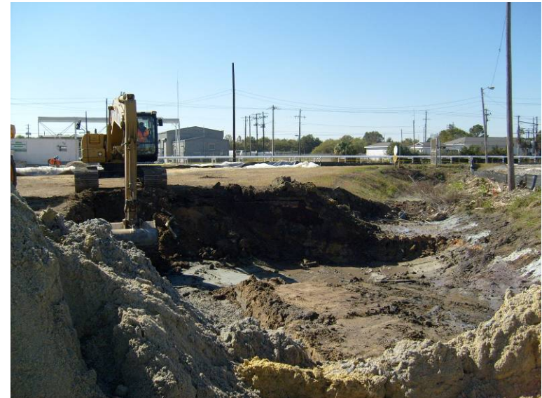
Photo 16: excavation in area A.
