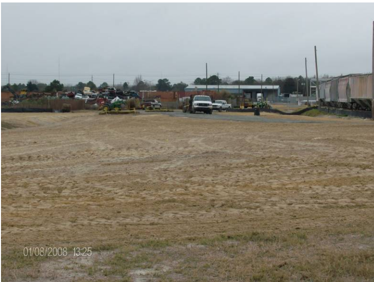
Photo 23: Final grade prior to seeding.
