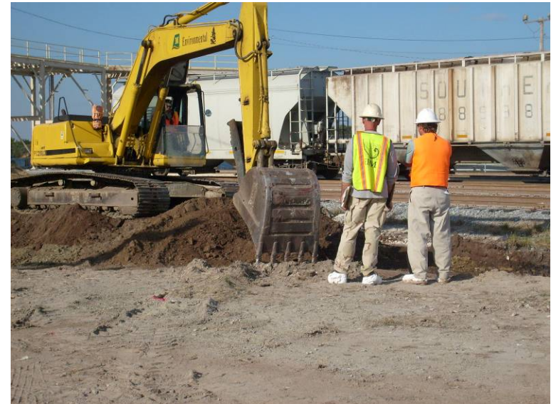
Photo 8: Excavation in area D.
