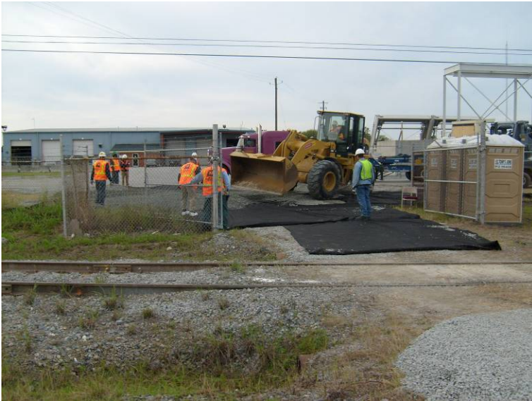
Photo 5: Erosion control installed at construction gate.
