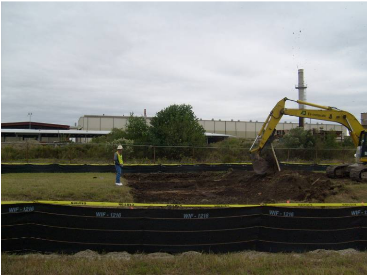
Photo 3: Excavation of area G.
