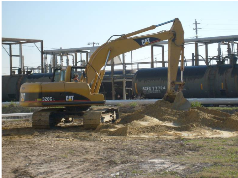
Photo 15: Backfill in area E.
