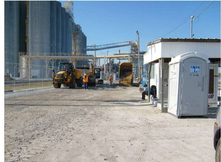
Photo 14: Backfill and restoration in area C.
