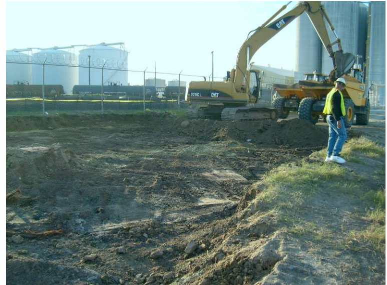
Photo 18: Excavation of area B-SUP.
