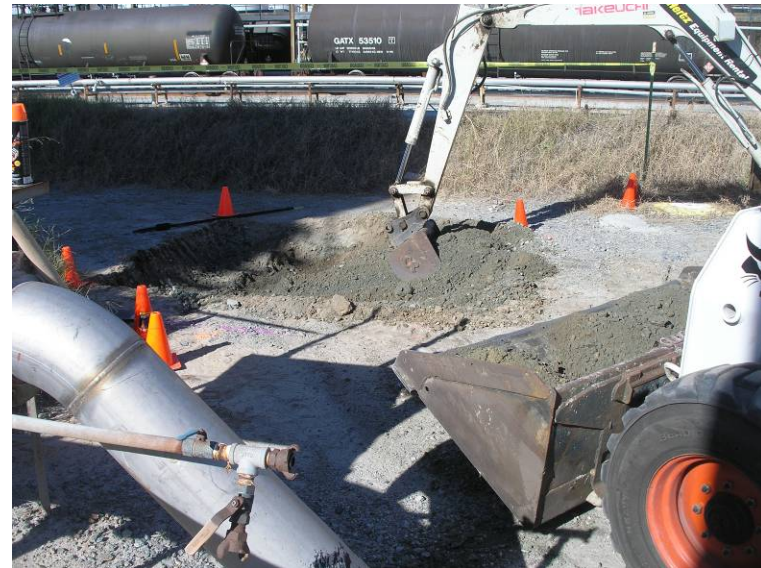
Photo 28: 2010 Area D during excavation.
