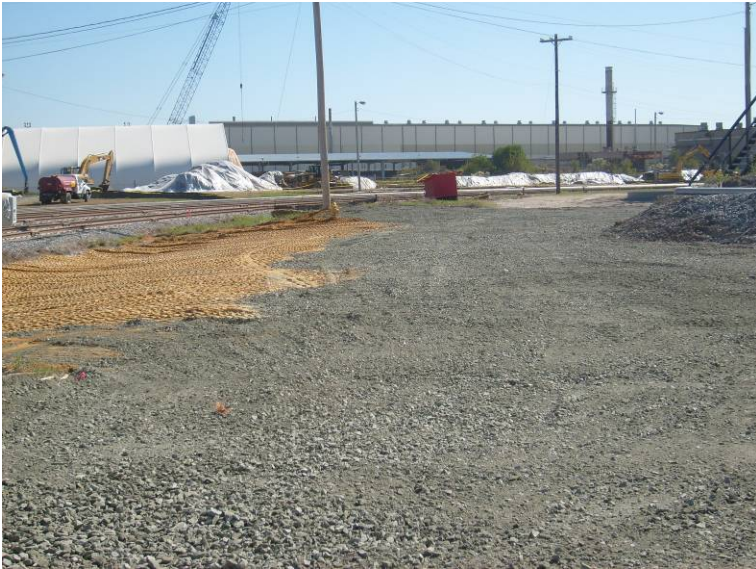
Photo 9: Area D completed.
