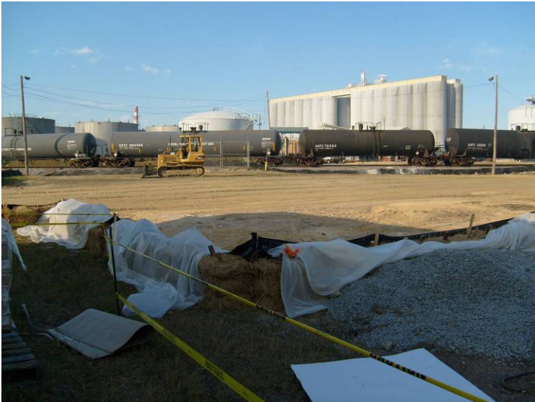
Photo 17: Restoration of area A.
