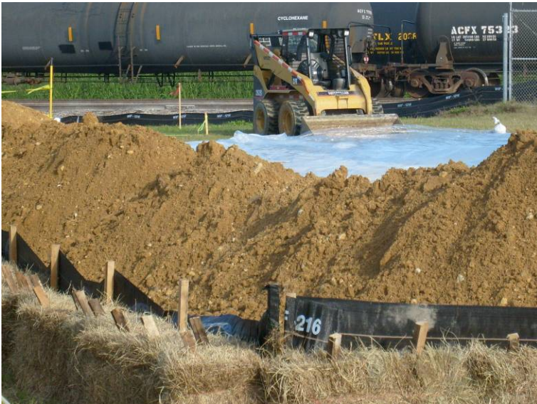
Photo 7: Clean backfill stockpile.
