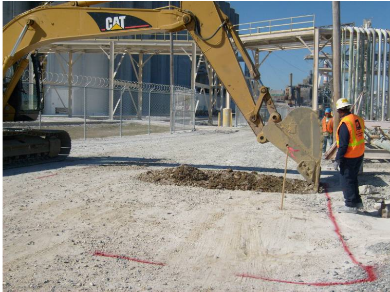
Photo 13: Excavation in area C.
