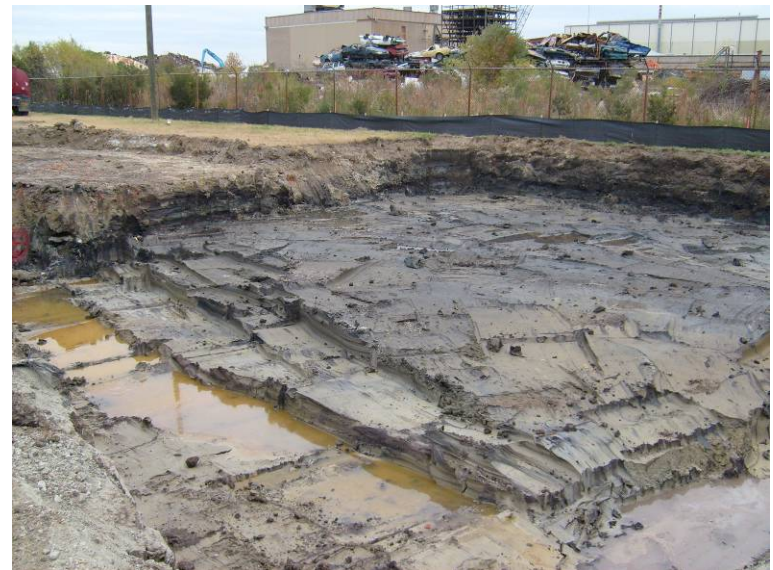
Photo 20: Excavation in area F.
