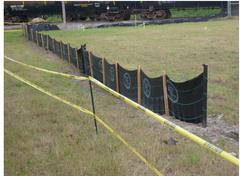
Photo 4: Installed silt fence.
