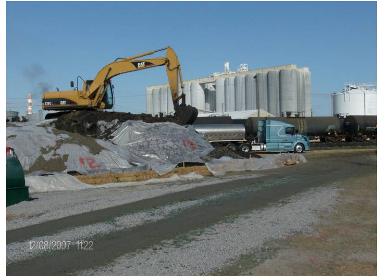
Photo 22: MAECTITE® application in SP-F3
