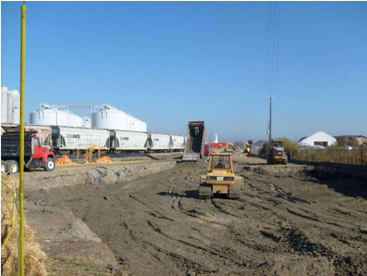
Photo 21: Backfill in area F.
