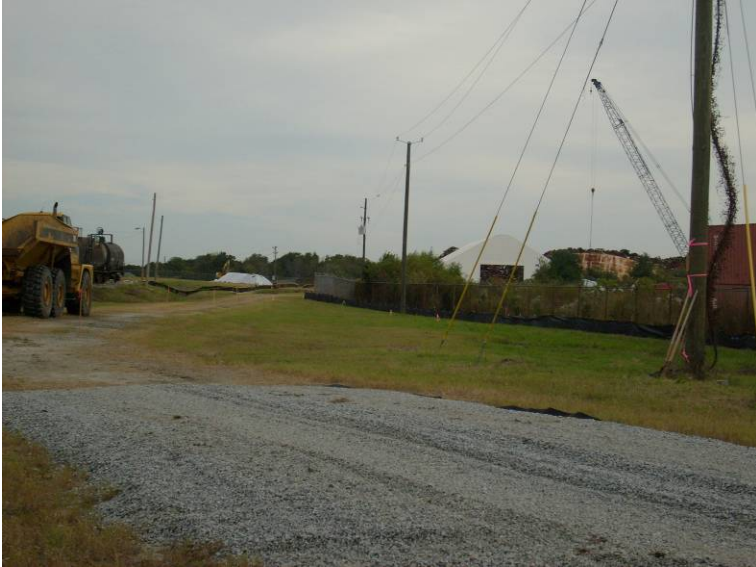
Photo 1: Site prior to excavation.
