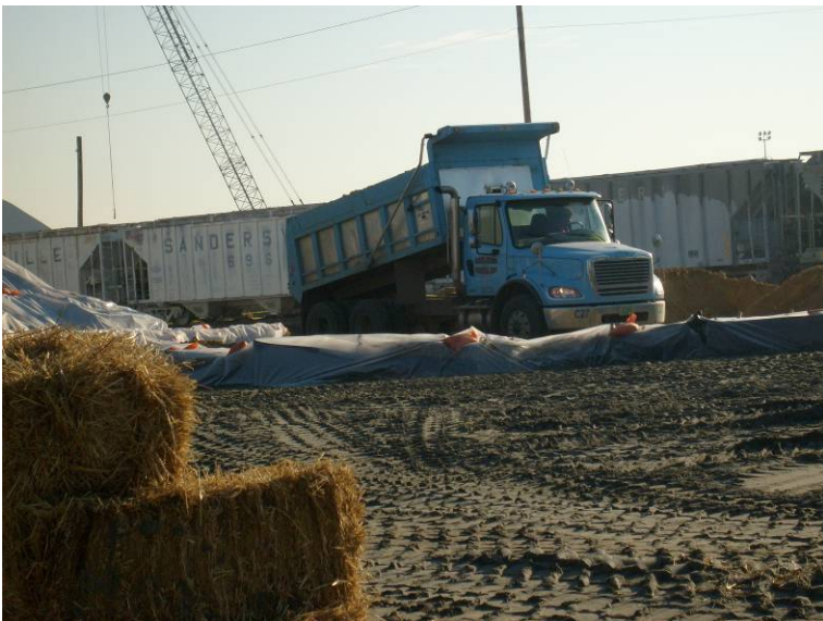
Photo 11: Backfill in area I.
