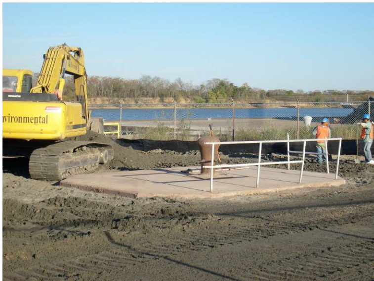
Photo 19: Backfill and restoration of area B-SUP.
