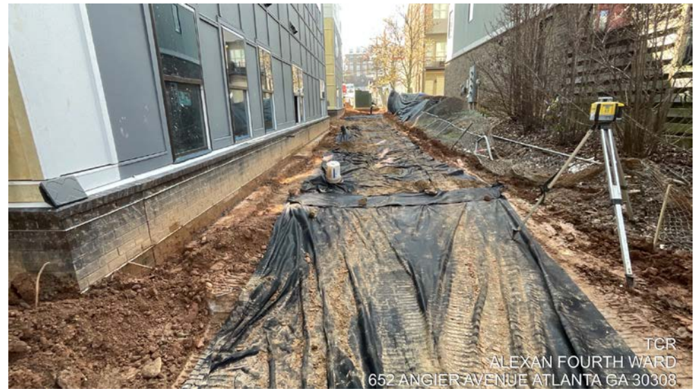
Photo: Witness barrier placement and rough-in staging
