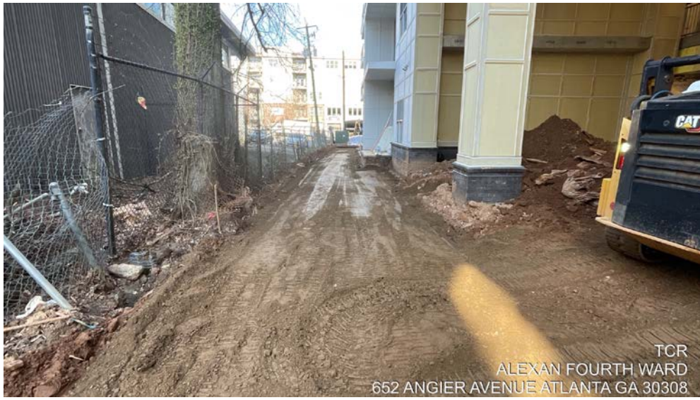
Photo: Placement and backfill of tested import soils atop witness barrier
