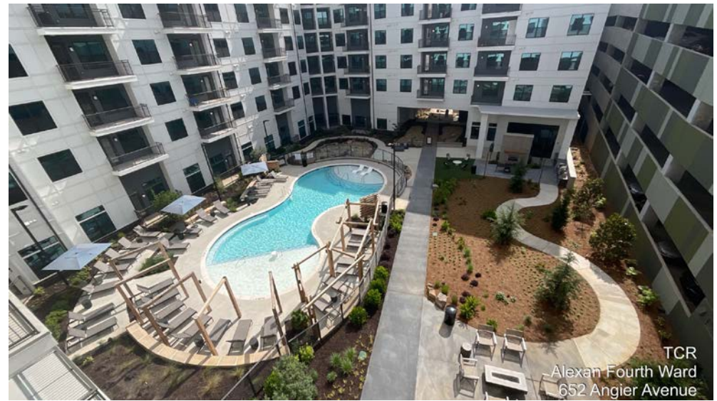
Photo: Final site conditions, interior courtyard/pool area
