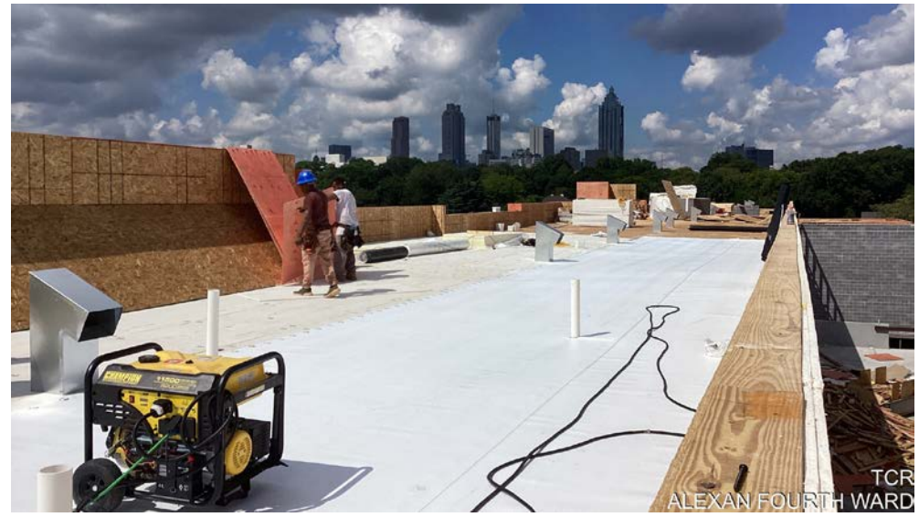
Photo: In-progress rooftop completion (including VIMS vents)
