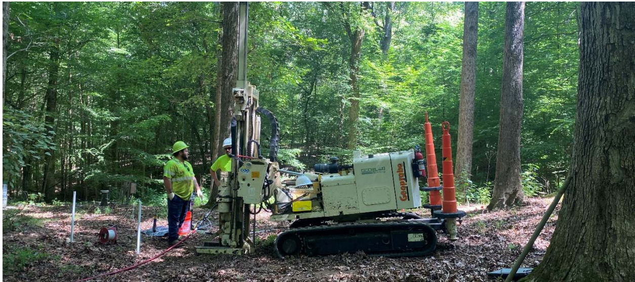
DPT Rig Injecting into the Subsurface
