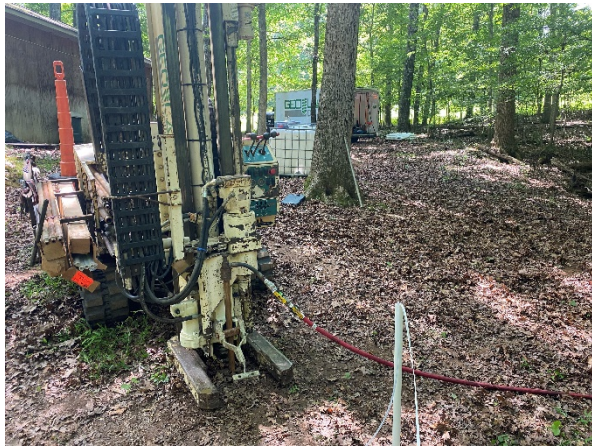
Injecting into the Subsurface
