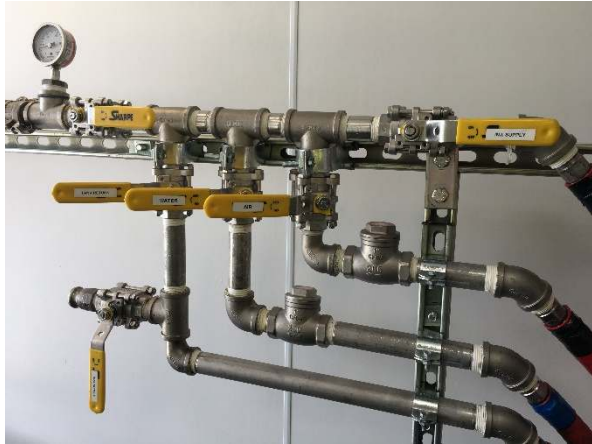
Stainless-steel Injection Manifold
