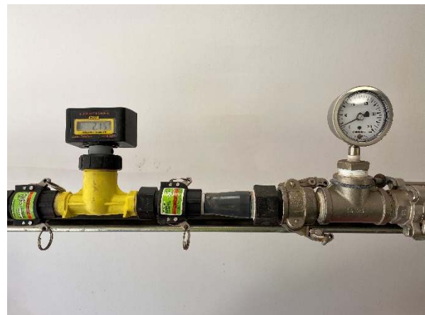
Monitoring Injection Flow and Pressure
