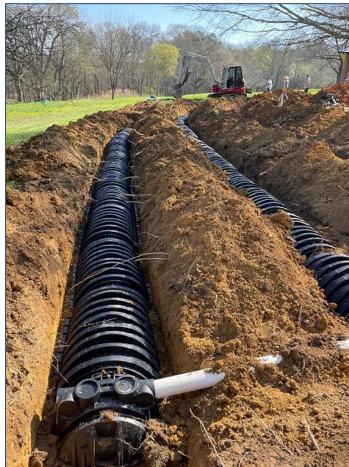
Figure 4: Example FY2019 Septic Repair BMP Project Installed in Pine Log and Salacoa Creek Watersheds
