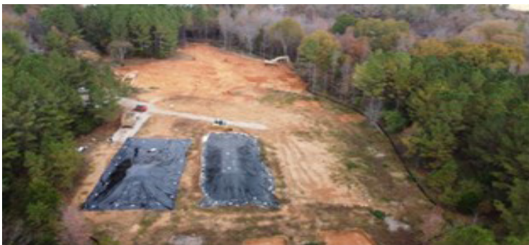
Cedartown Battery Site (HSI No. 10106): View of excavation areas.
