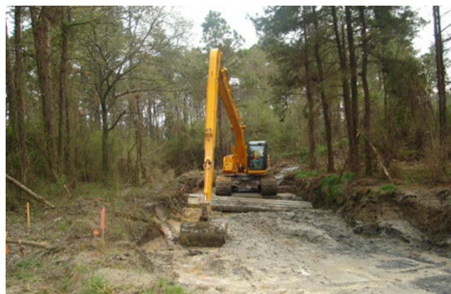
HTWP Stream channel excavation (HSI# 10199).
