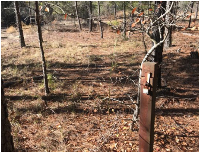
Monitoring well at Palmetto Tire Fire Site, HSI 10327, Coweta County
