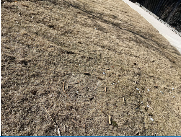
Photo 1: Soil cap cover and planted vegetation above soil nail wall.
