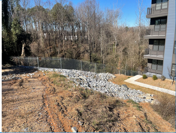
Photo 2: Rip rap embankment west of soil cap cover.
