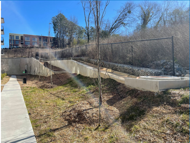
Photo 3: Soil nail wall south of development.
