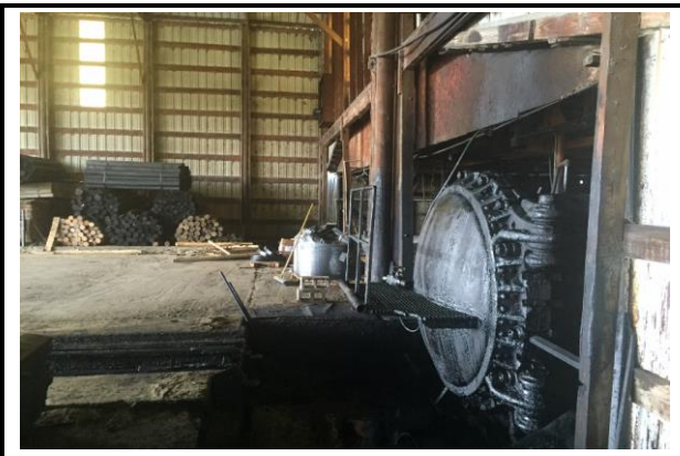
View: Creosote Retort at the central portion of the facility
