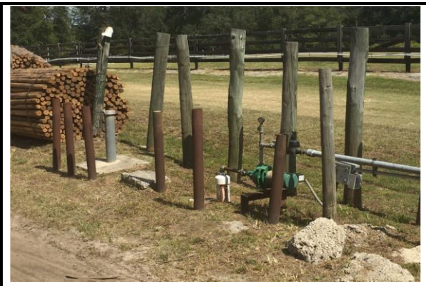
View: Recovery well outside of impoundment
