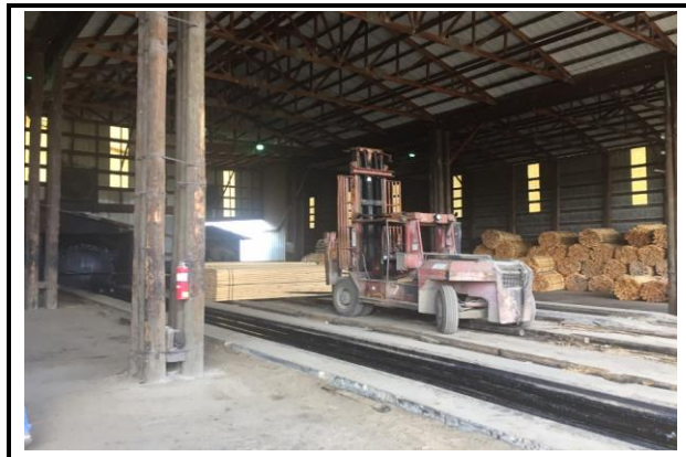
View: The interior drying shed for treated poles at the central portion of the facility.
