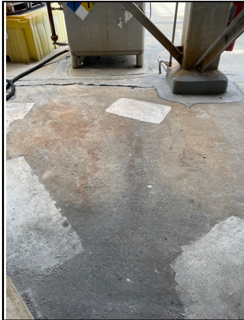
Former PCE Drum Area
