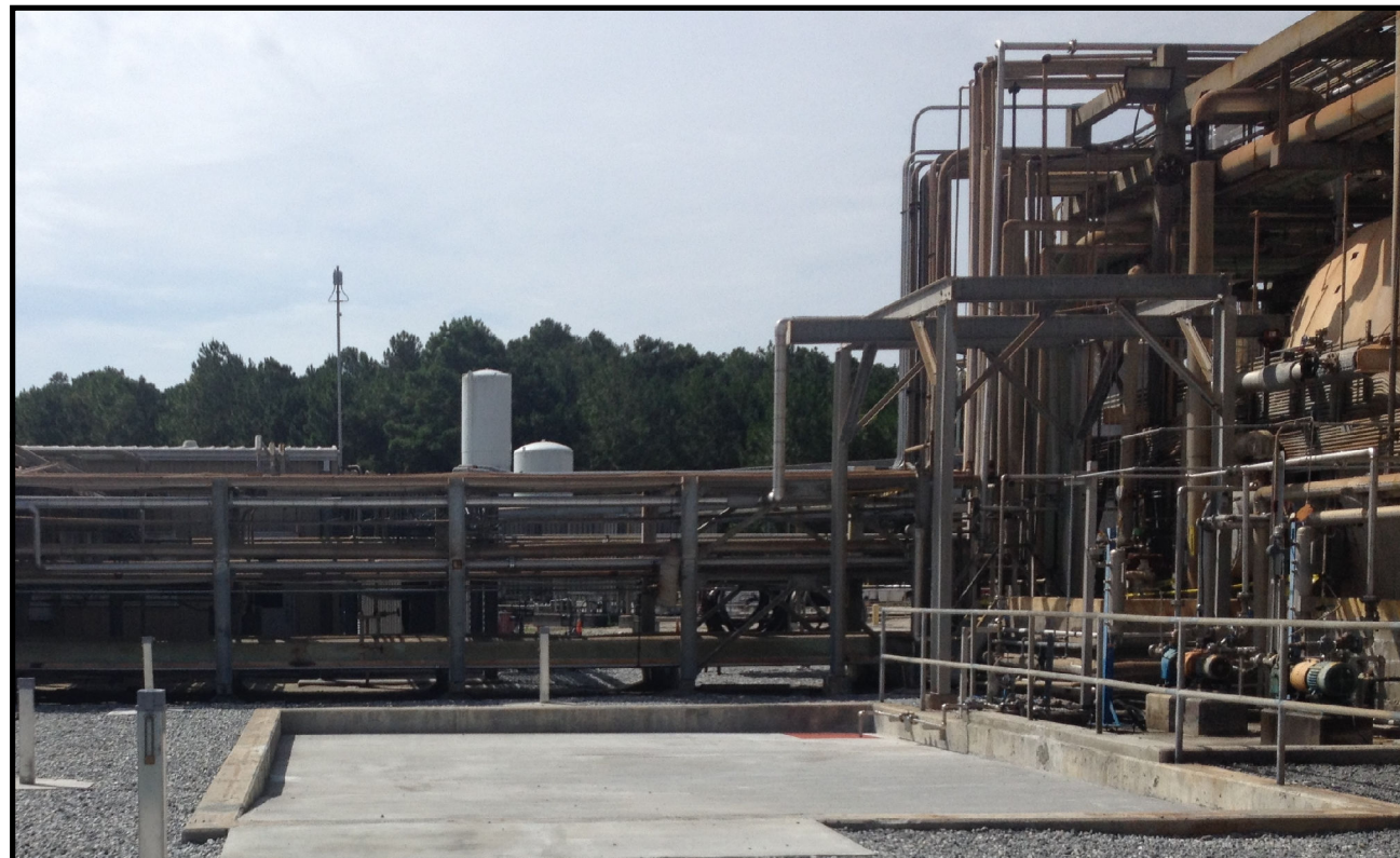
Former First Flush Basin
