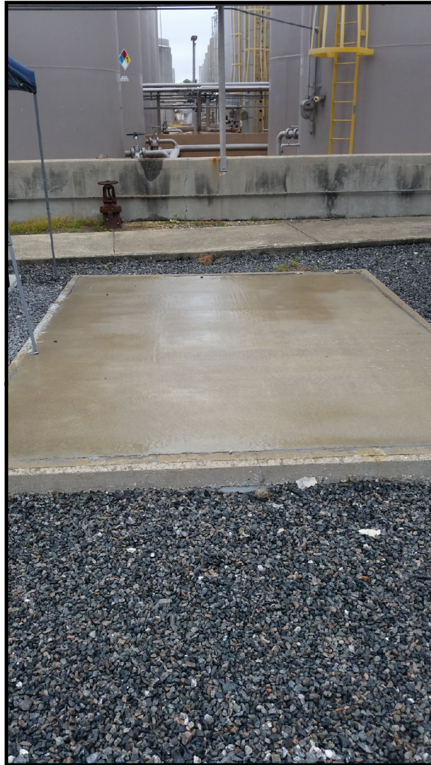
Former Process Wet Well
