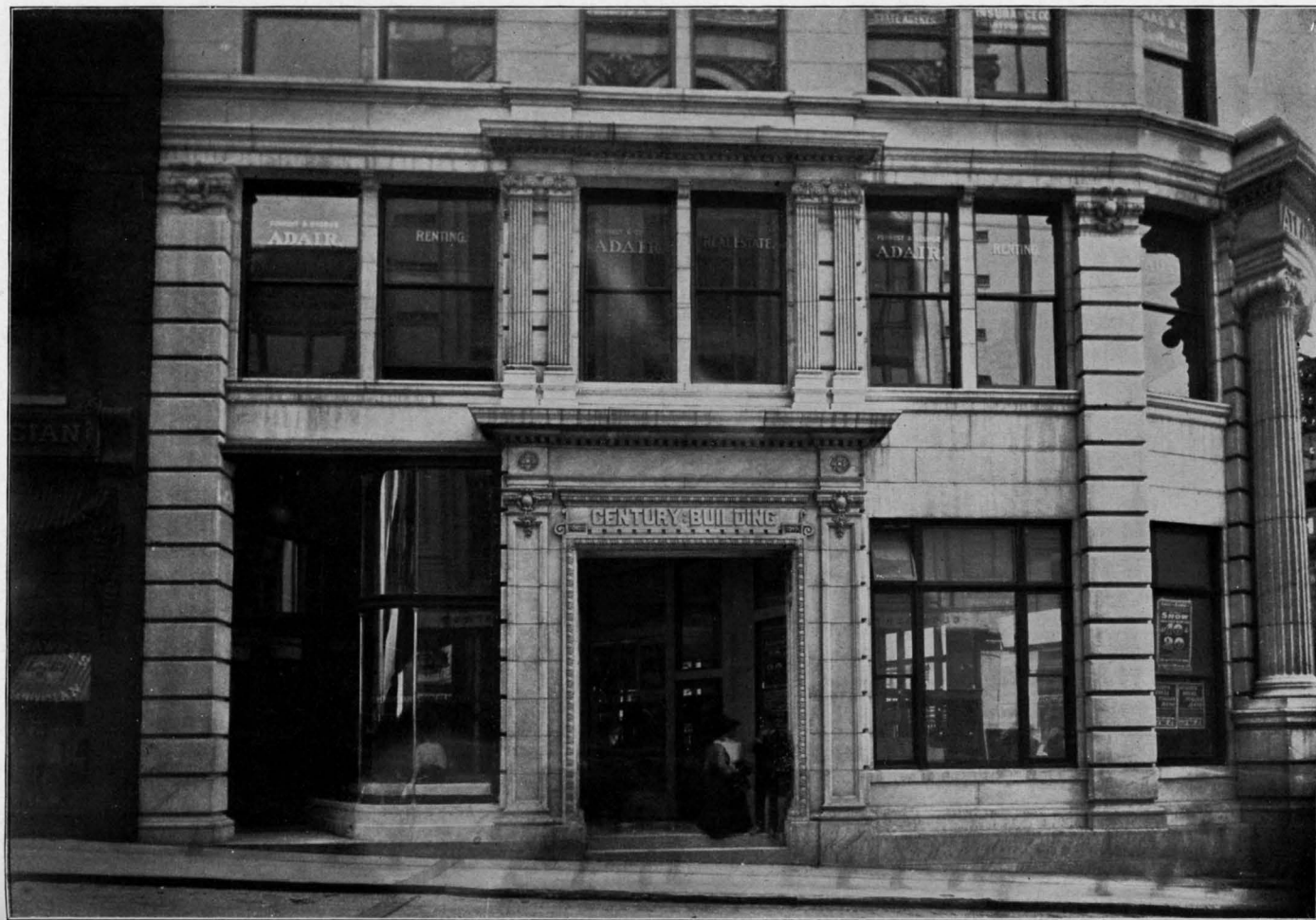
ENTRANCE TO THE CENTURY OFFICE BUILDING, ATLANTA, GEORGIA. THE FIRST FOUR STORIES CONSTRUCTED OF WHITE GEORGIA MARBLE BY THE BLUE RIDGE MARBLE COMPANY, NELSON, GEORGIA.
