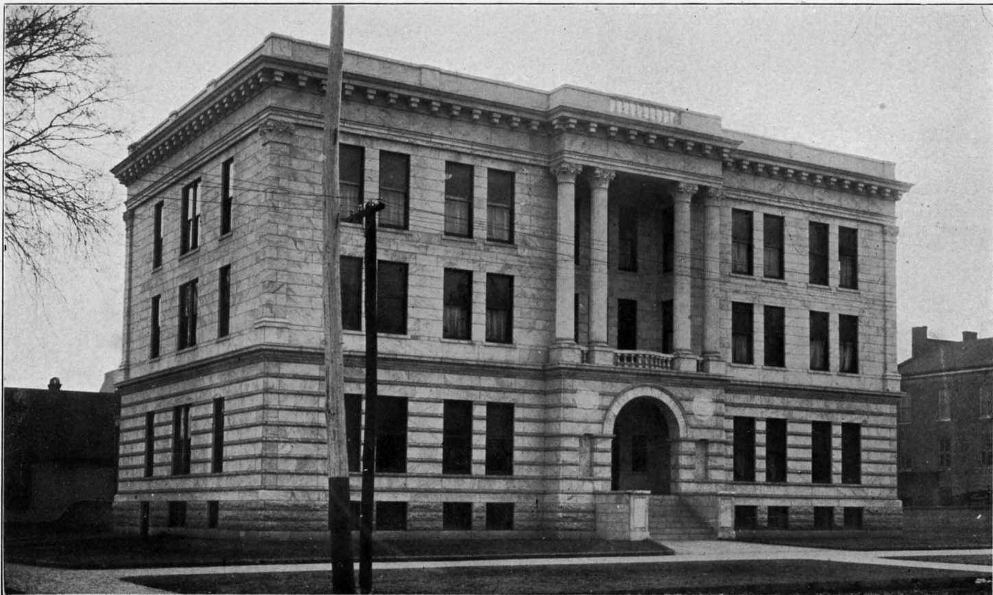
THE YOUNG MEN'S CHRISTIAN ASSOCIATION BUILDING, COLUMBUS, GEORGIA. BUILT OF GEORGIA MARBLE BY THE BLUE RIDGE MARBLE COMPANY, NELSON, GEORGIA.
