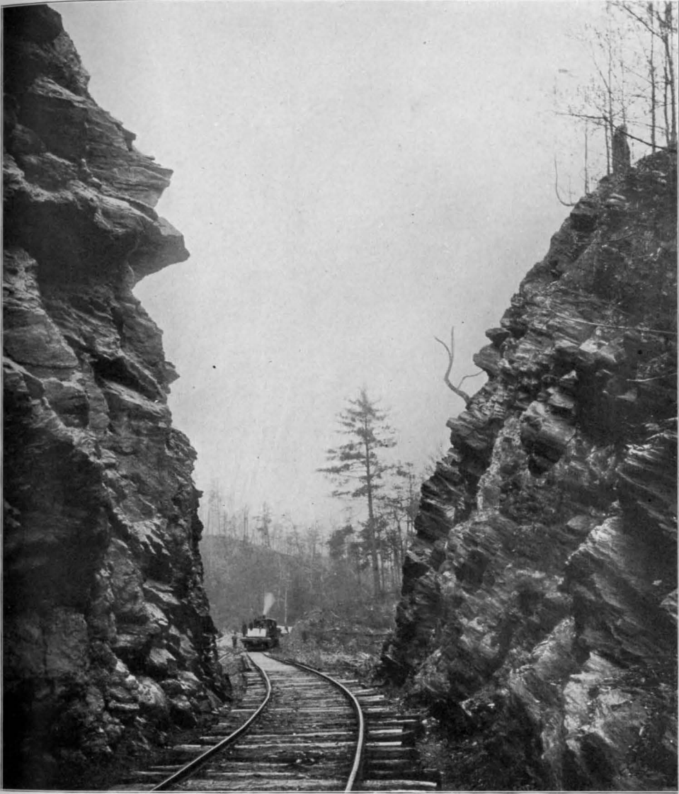
A CUT ALONG THE AMICALOLA RAILROAD, SHOWING THE COUNTRY ROCK (MICA-SCHIST) OF THE MARBLE DEPOSITS OF PICKENS COUNTY, GEORGIA.
