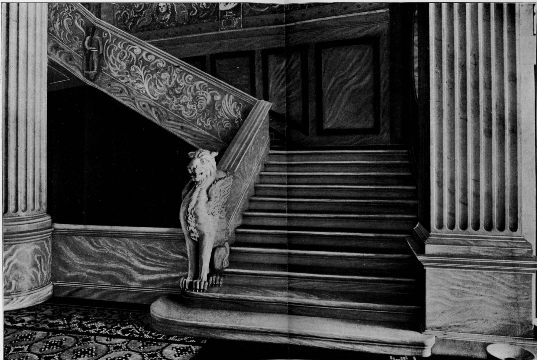
MARBLE COLUMNS AND STAIRCASE IN THE BASEMENT OF THE CANDLER BUILDING, ATLANTA, GEORGIA, SHOWING CARVINGS IN GEORGIA MARBLE, FROM THE AMICALOLA MARBLE QUARRIES, PICKENS COUNTY, GEORGIA.
