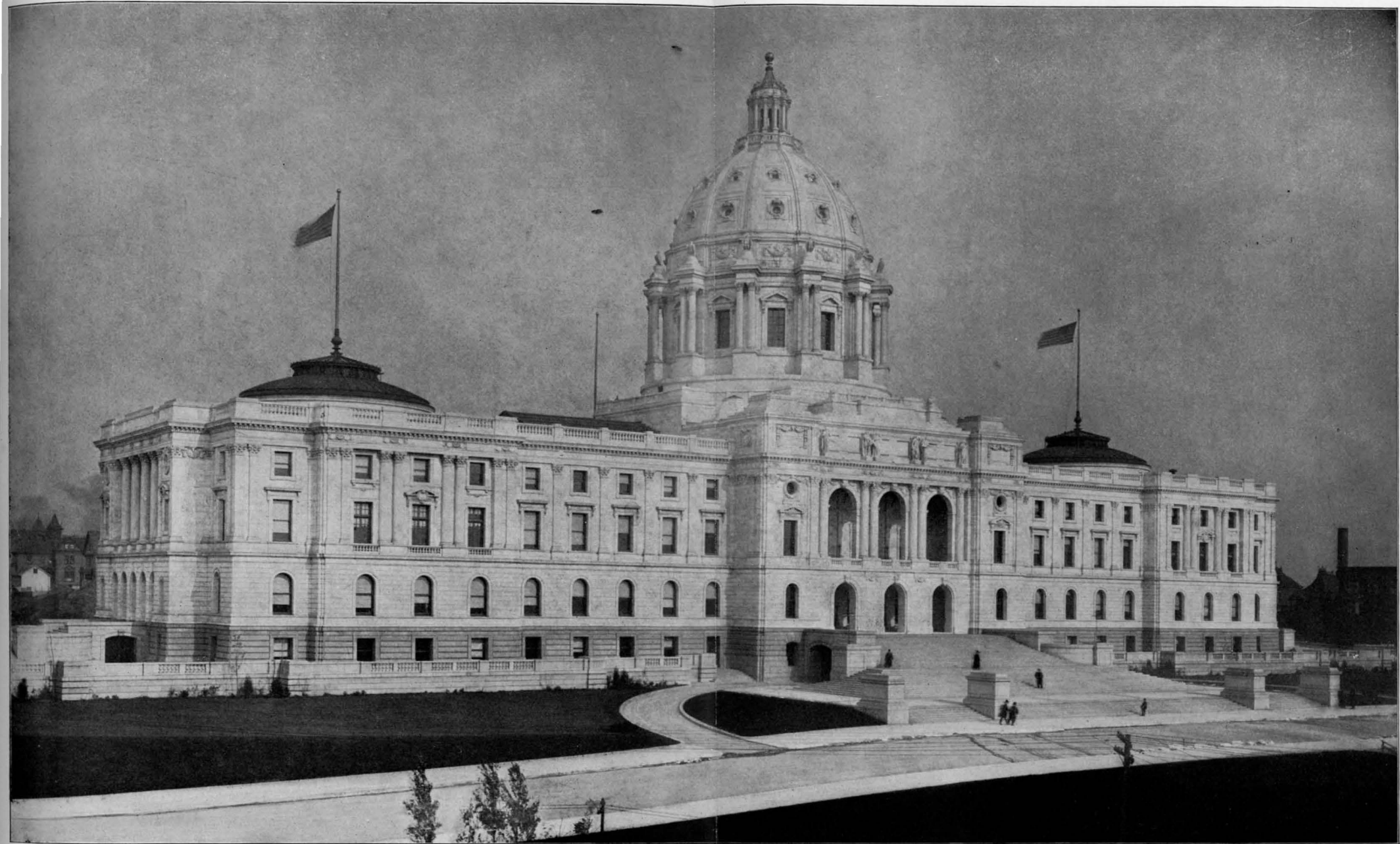
MINNESOTA STATE CAPITOL, ST. PAUL, MINN. BUILT OF WHITE GEORGIA MARBLE FROM THE AMICALOLA QUARRIES, PICKENS COUNTY, GEORGIA.
