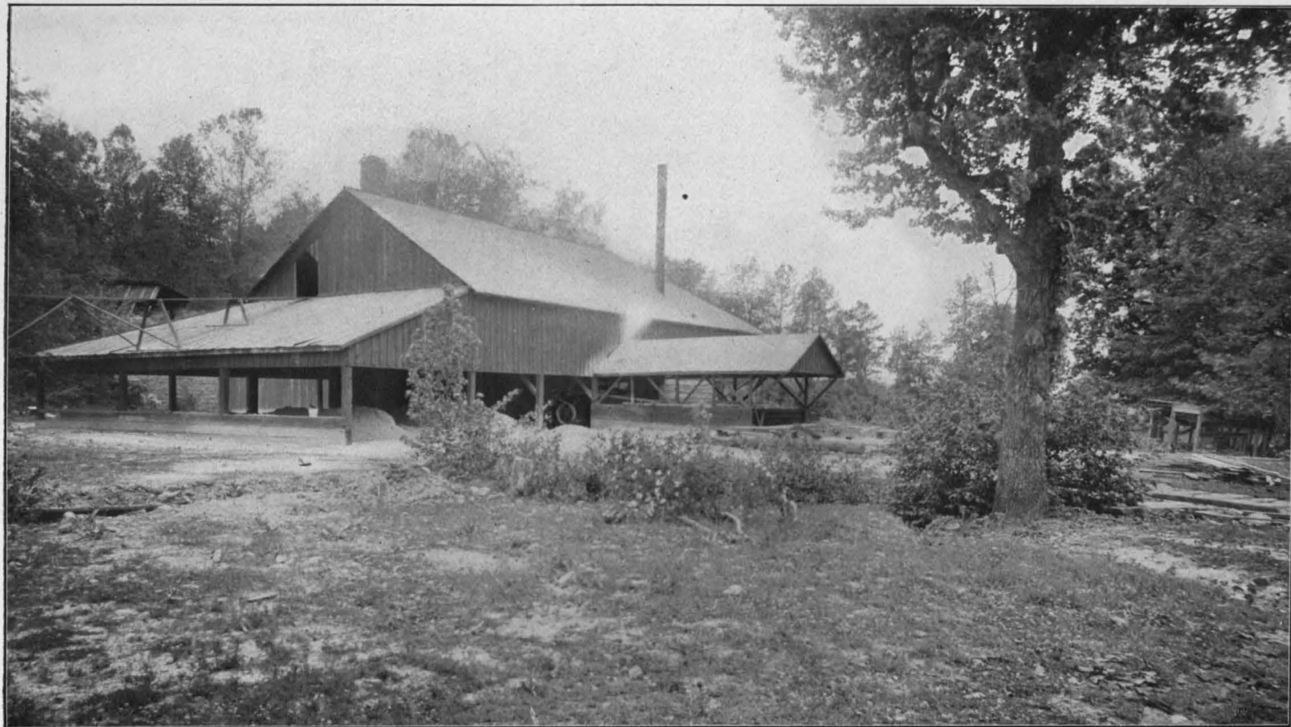
GENERAL VIEW OF THE BAUXITE DRYING PLANT OF THE REPUBLIC MINING AND MANUFACTURING COMPANY, HERMITAGE, FLOYD COUNTY, GEORGIA.
