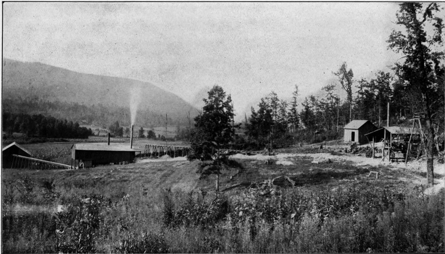
GENERAL VIEW OF THE GULLIVER BAUXITE PLANT, WALKER COUNTY, GEORGIA.
