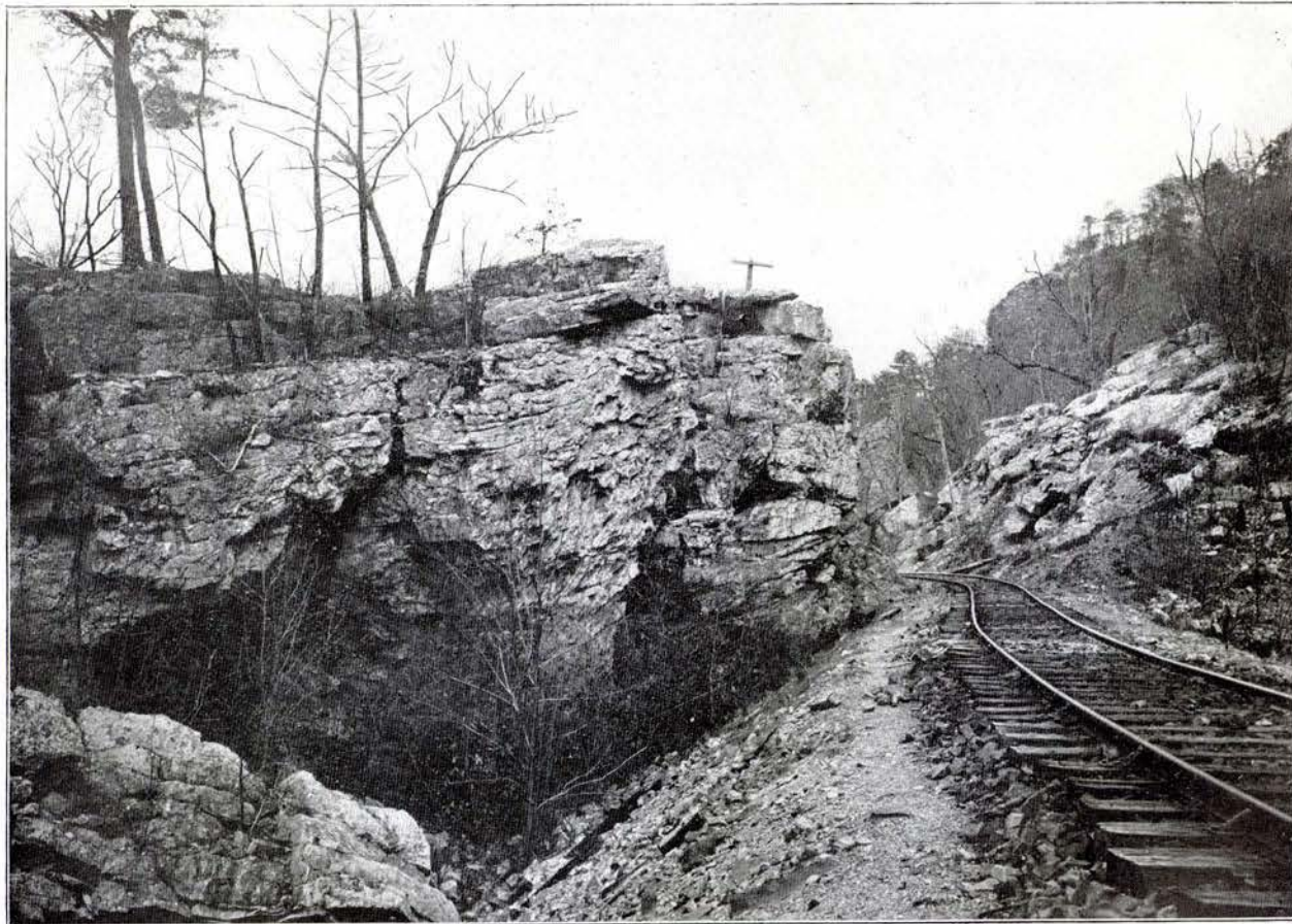
CUT ALONG THE DURHAM RAILROAD, NEAR LULA LAKE, WALKER COUNTY, GEORGIA, SHOWING AN EXPOSURE OF LOOKOUT SANDSTONE.
