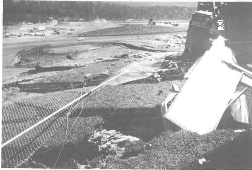
Figure 10 - Shifted joint blocks of deeply weathered, fine-grained sandstone and siltstone on east side of damaged apartment (numbered 2 in Figure 4) two days after initial movement. View looking southeast across Festival Centre terrace under construction. Photograph by M. J. Neilson.
