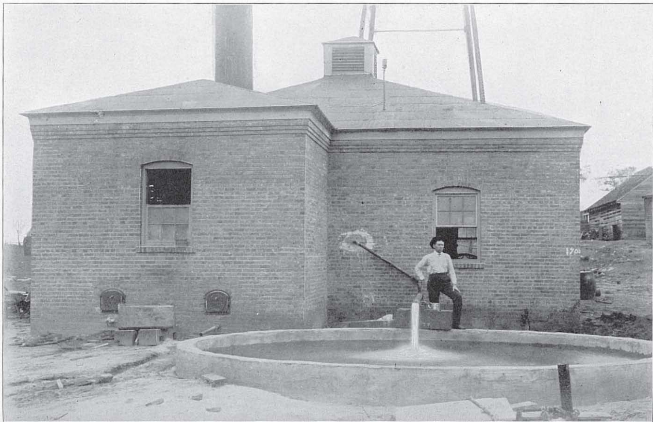
RESERVOIR AND PUMPING STATION AT THE BLAKELEY DEEP WELL, BLAKELEY, EARLY COUNTY, GEORGIA.
