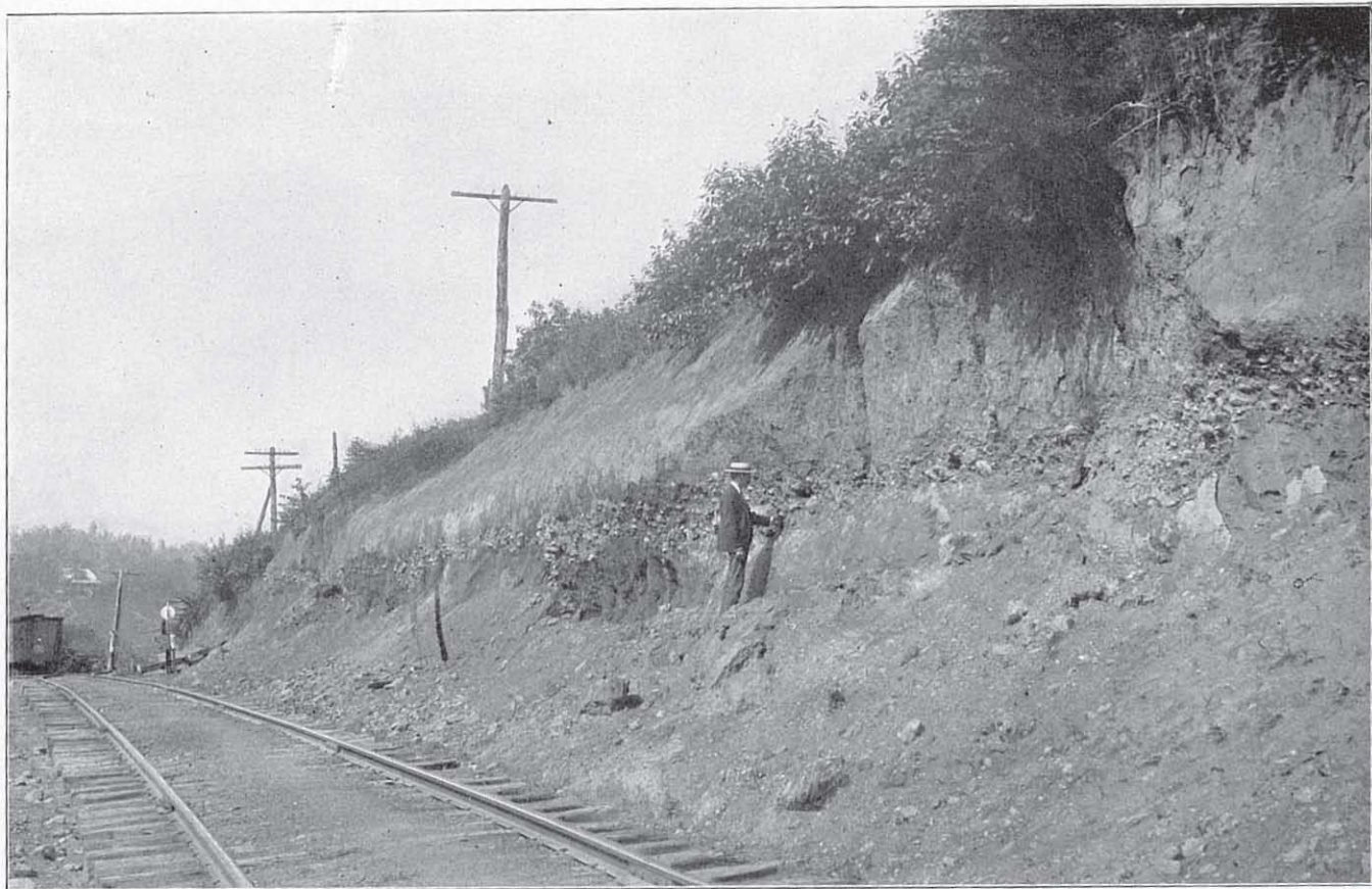
CUT ALONG THE LOUISVILLE & NASHVILLE RAILROAD AT ELIJAY, GILMER COUNTY, GEORGIA, SHOWING SECTION OF THE ALLUVIAL DEPOSITS, WHICH SUPPLY THE SHALLOW WELLS OF THE TOWN WITH WATER.
