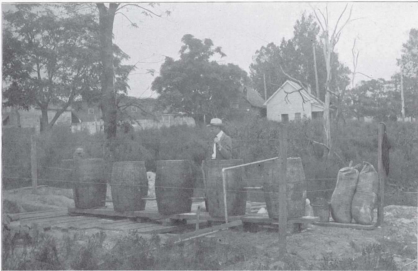
VIEW SHOWING HOW SALT WAS INTRODUCED IN THE WELL, DURING THE QUITMAN EXPERIMENT.
