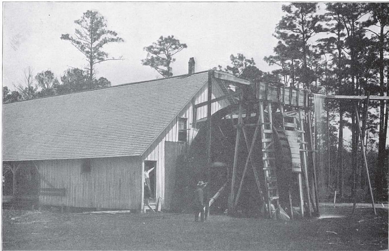
A RICE MILL AT TARBORO, CAMDEN COUNTY, GEORGIA, OPERATED BY ARTESIAN WELLS.
