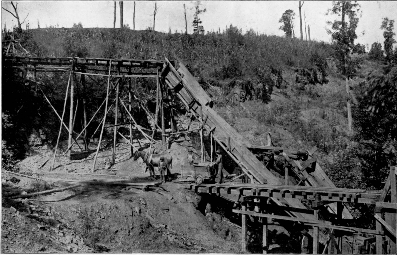
THE DOUBLE TIPPLE, KENSINGTON IRON AND COAL COMPANY'S PROPERTY, NEAR ESTELLE, WALKER COUNTY, GEORGIA.
