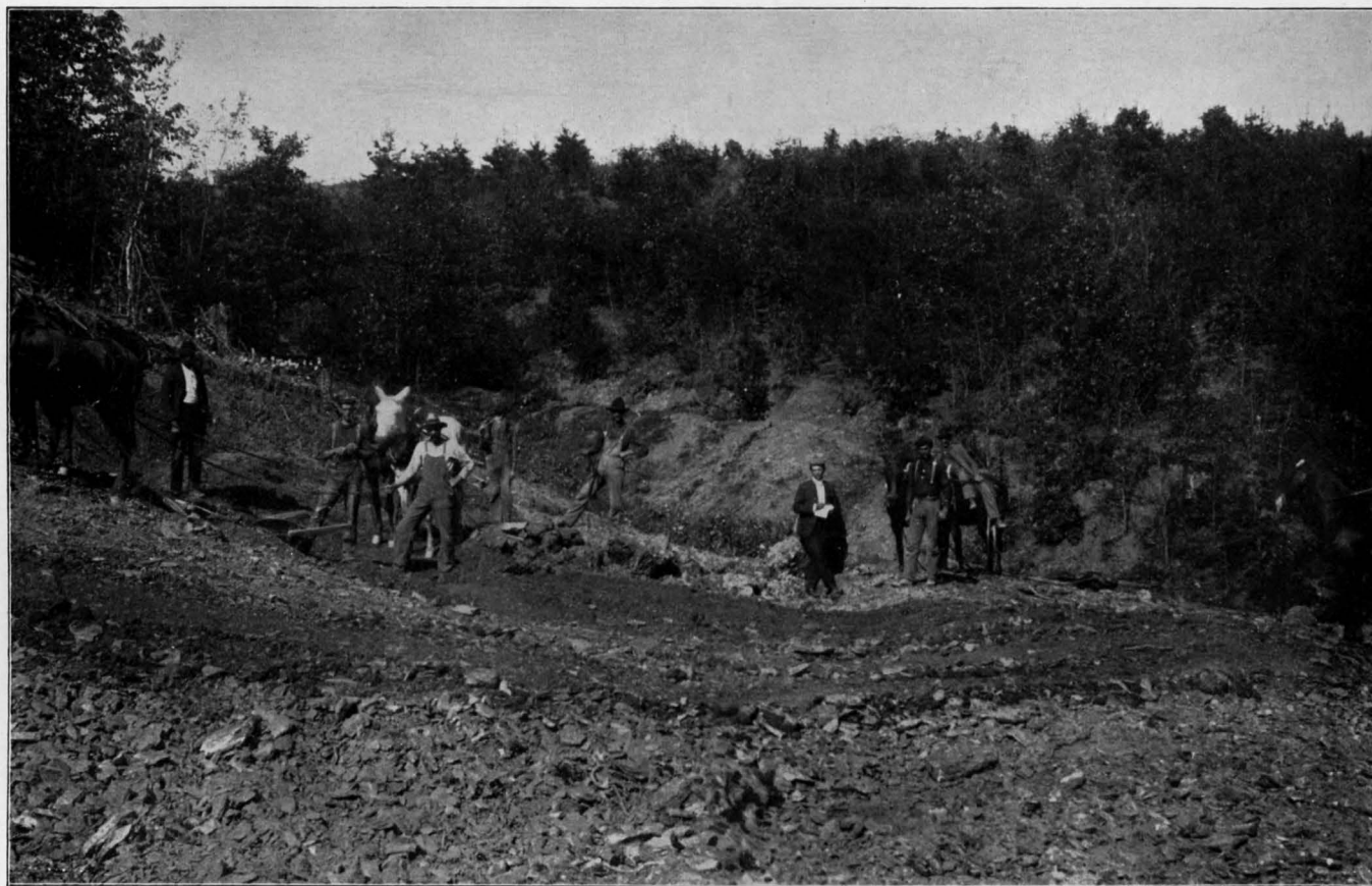
MINING FOSSIL IRON ORE BY SURFACE STRIPPING ON THE KENSINGTON IRON AND COAL COMPANY'S PROPERTY, NEAR ESTELLE, WALKER COUNTY, GEORGIA.
