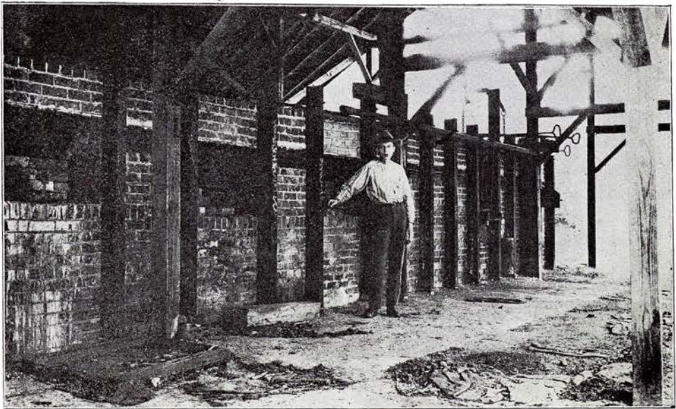
FIG. 2.—VIEW OF A PORTION OF ROASTING AND SMELTING FURNACE, SEMINOLE GOLD AND COPPER MINE, LINCOLN COUNTY, GEORGIA
