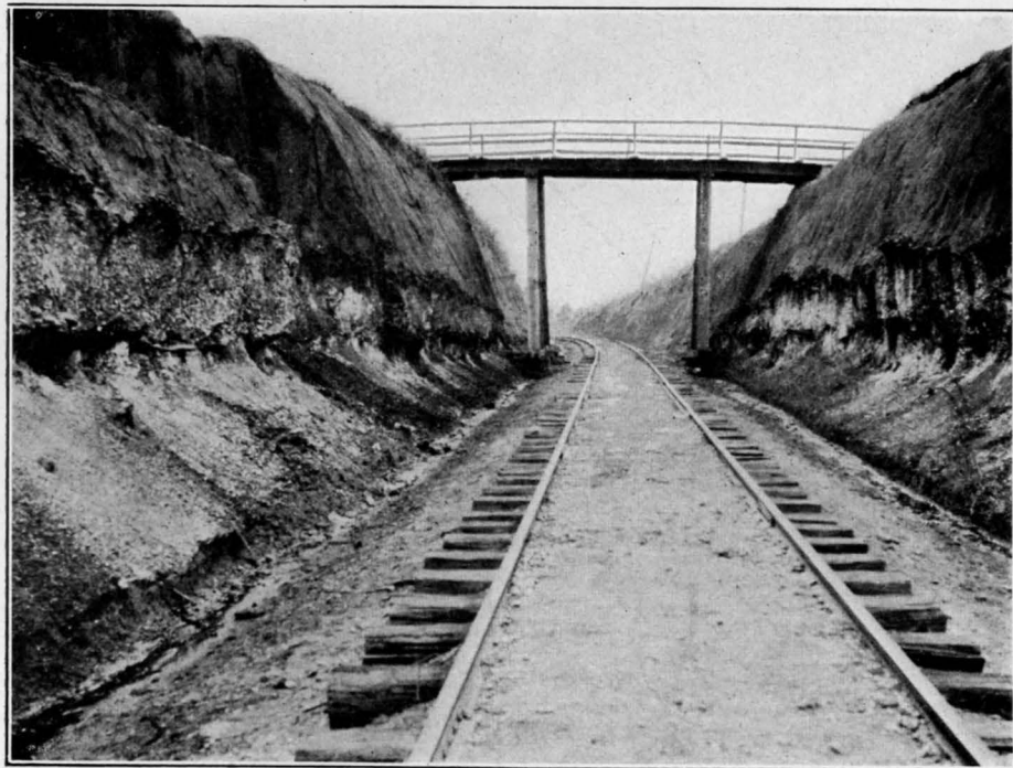
B. CUT OF C. OF GA. RY., ONE MILE SOUTHEAST OF BUENA VISTA, SHOWING UNCONFORMABLE CONTACT BETWEEN PROVIDENCE SAND MEMBER OF THE RIPLEY AND OVERLYING EOCENE.
