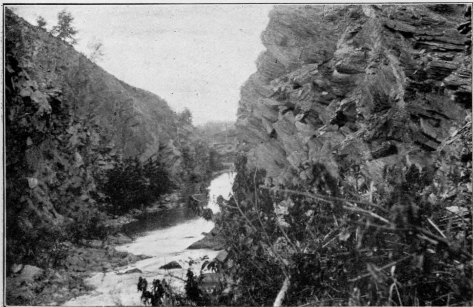
B. ROCKMART SLATES. ARTIFICIAL CUT MADE BY SEABOARD RAILROAD IMMEDIATELY SOUTH OF ROCKMART, POLK COUNTY, GEORGIA
