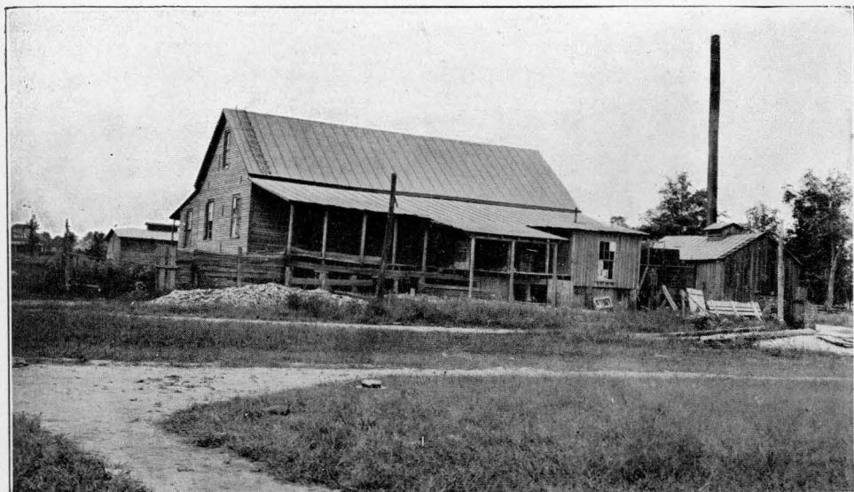
A. COHUTTA TALC COMPANY'S MILL, CHATSWORTH, MURRAY COUNTY.
