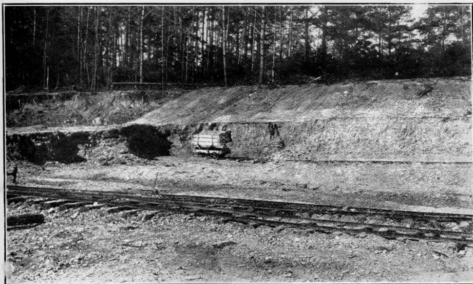
B. WORKING FACE IN THE FULLERS EARTH MINE OF THE LESTER CLAY CO., ATTAPULGUS, DECATUR COUNTY.
