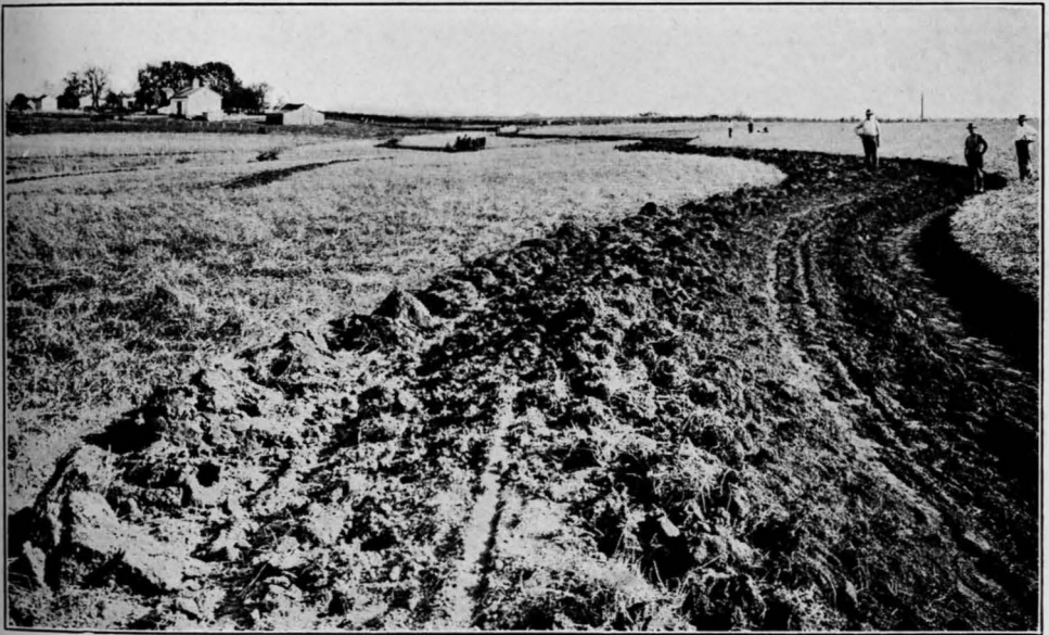
B. RIDGE TERRACE UNDER CONSTRUCTION
