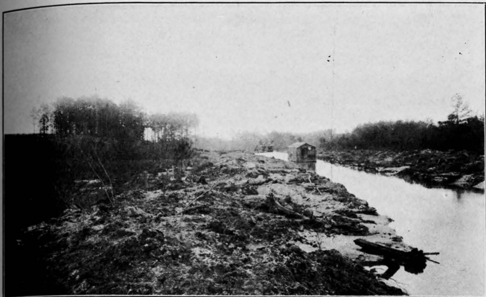
A. DITCH UNDER CONSTRUCTION, BIG HAYNES CREEK, GWINNETT COUNTY, GEORGIA
