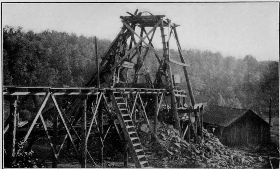
B. LITTLE BOB PYRITE MINE, PAULDING COUNTY. CLOSE VIEW OF HEAD-FRAME AND PICKING FLOOR.
