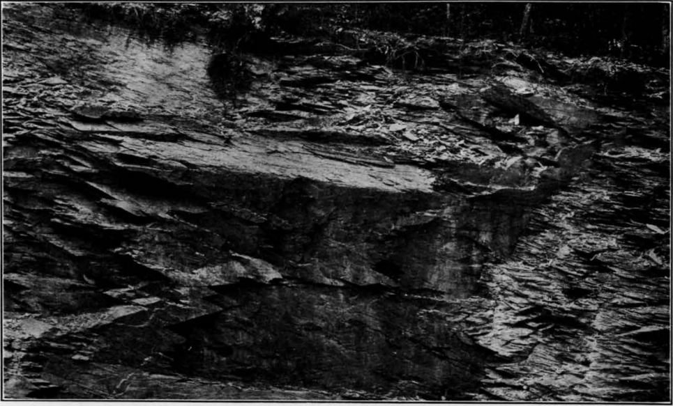
A. QUARRY OF THE GEORGIA GREEN SLATE COMPANY NEAR BOLIVAR, BARTOW COUNTY, SHOWING THE EXTENSIVE JOINTING WHICH MADE WORKING DIFFICULT.
