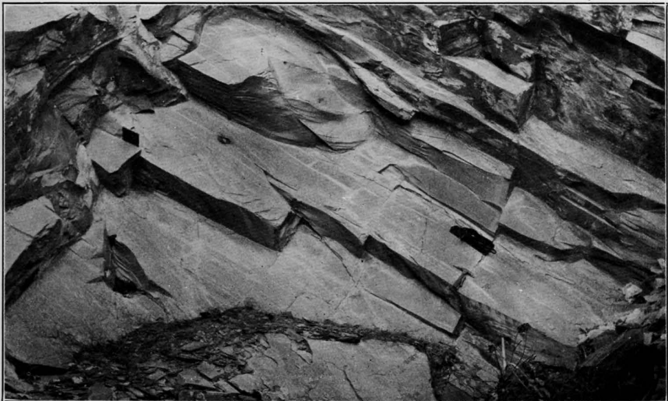
B. OLD DEVER QUARRY, ROCKMART, POLK COUNTY, SHOWING PROMINENT JOINTS ALMOST PERPENDICULAR TO THE CLEAVAGE. THE NOTE BOOK STANDS PARALLEL TO THE PRINCIPAL JOINT PLANES.
