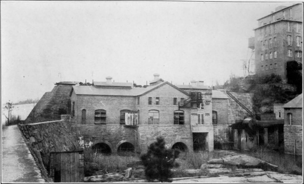
POWER PLANT AND DAM, NORTH HIGHLANDS DEVELOPMENT, COLUMBUS POWER COMPANY, CHATTAHOOCHEE RIVER NEAR COLUMBUS, GEORGIA.
