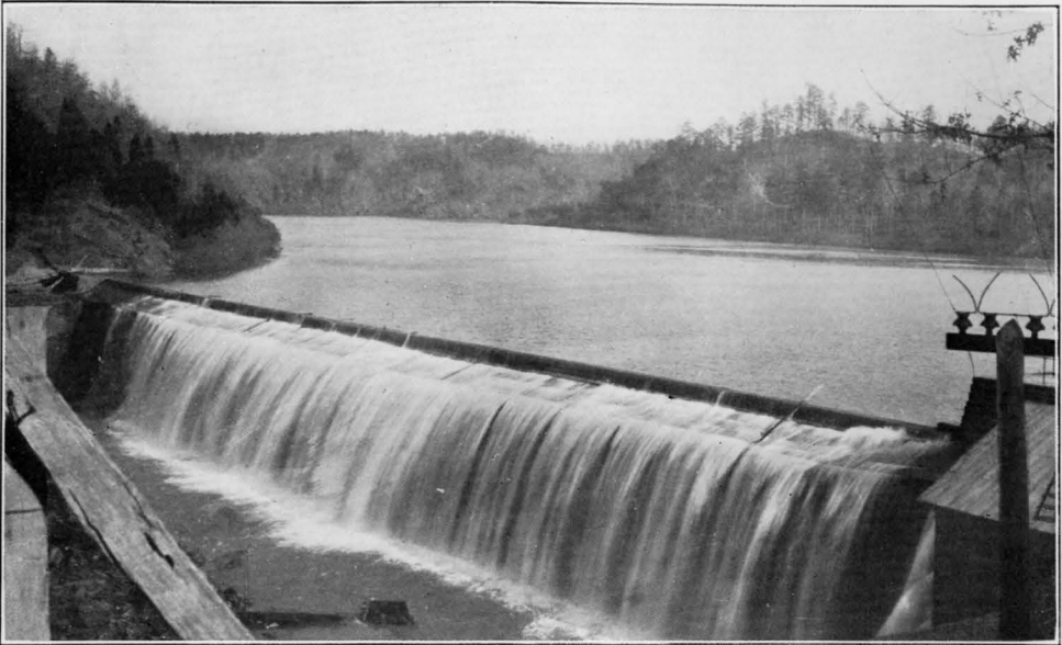
DAM, DUNLAP SHOALS, GEORGIA RAILWAY & POWER COMPANY, CHATTAHOOCHEE RIVER NEAR GAINESVILLE, GEORGIA.
