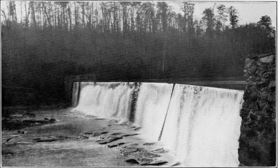
DAM, MITCHELL'S BRIDGE, ATHENS RAILWAY & ELECTRIC COMPANY, OCONEE RIVER NEAR ATHENS, GEORGIA.
