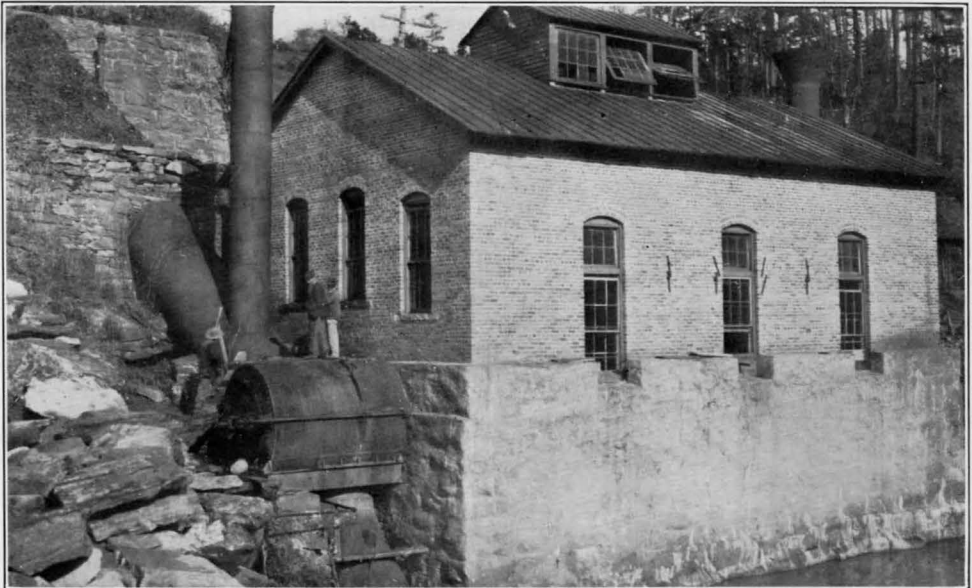
TALLASSEE SHOALS POWER PLANT, ATHENS RAILWAY & ELECTRIC COMPANY, OCONEE RIVER, NEAR ATHENS, GEORGIA.
