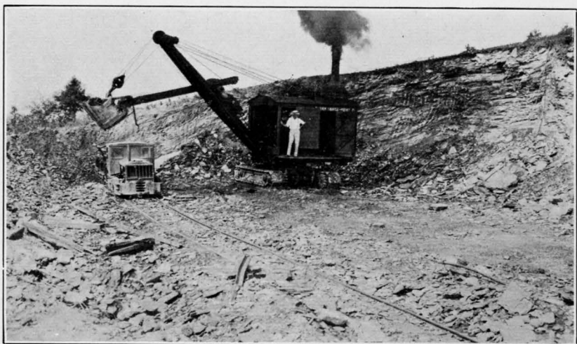
B. SHALE PIT OF THE PLAINVILLE BRICK COMPANY, PLAINVILLE, GORDON COUNTY.
