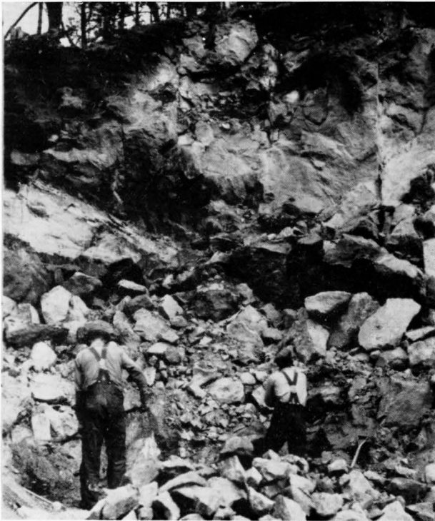
FIGURE B.—Screening out fines in olivine quarry after blast.
