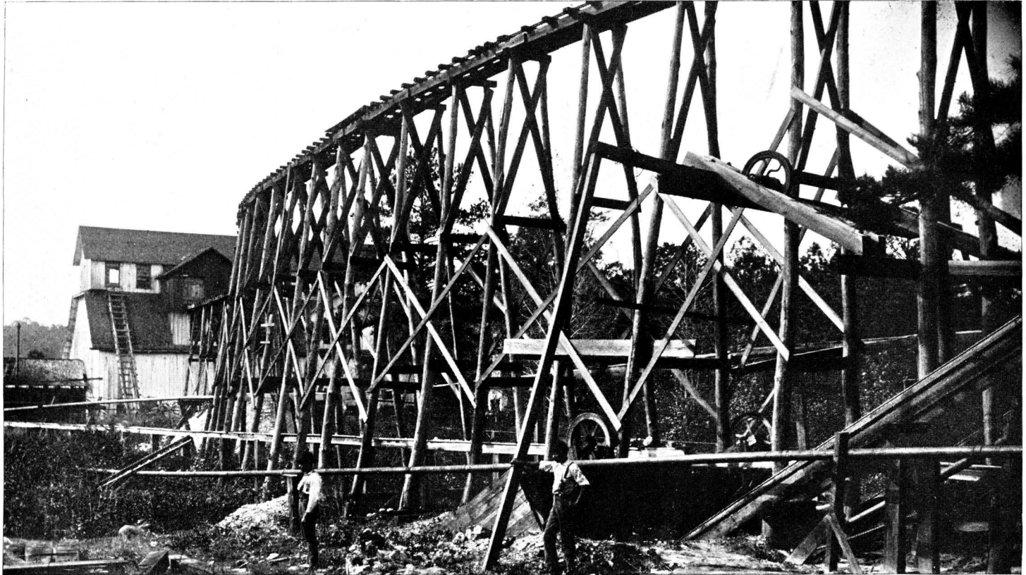
THE ROYAL GOLD MINE AND MILL, NEAR TALLAPOOSA, HARALSON COUNTY GEORGIA, SHOWING INCLINED AND ELEVATED RAILROAD, *USED FOR CONVEYING ORE FROM MINE TO MILL.
