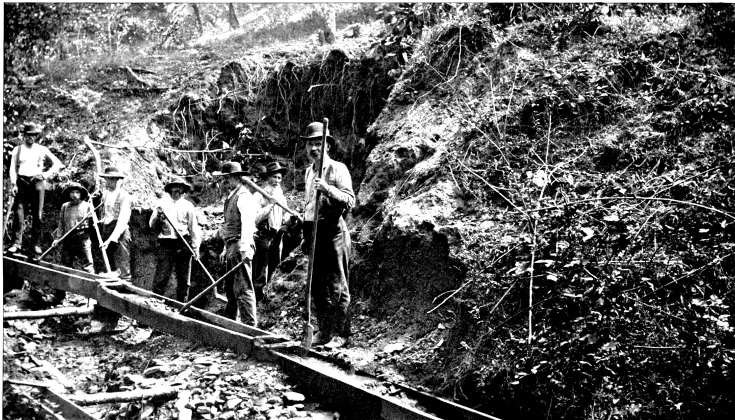
PLACER-MINING AT THE NEWTON GOLD-MINE, TOWNS COUNTY, GEORGIA.
