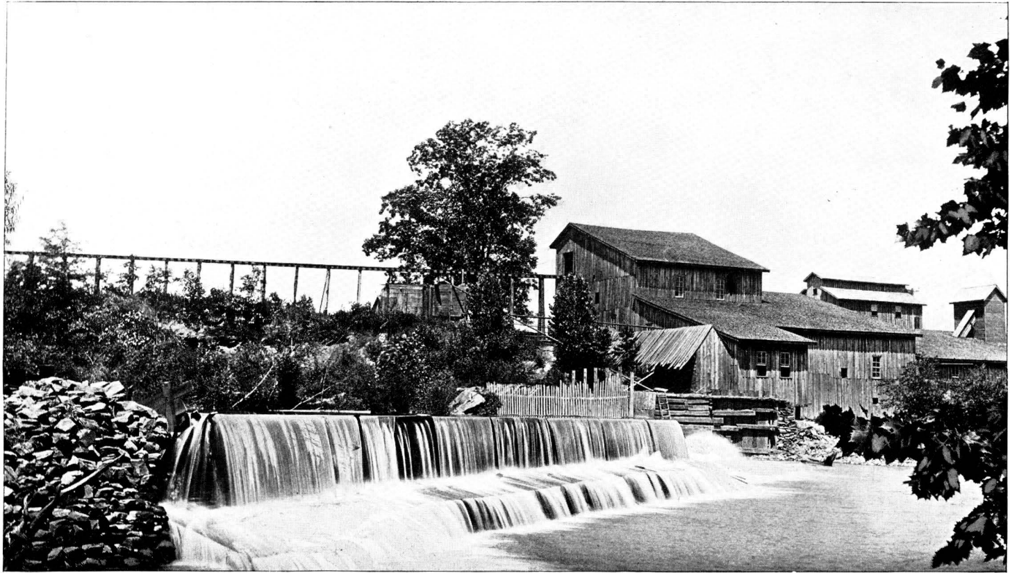
STAMP-MILL AND DAM ACROSS THE ETOWAH RIVER, CREIGHTON GOLD MINE, CHEROKEE COUNTY GEORGIA.
