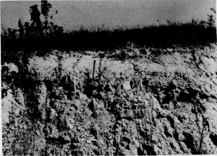
FIGURE 2. Road cut on old Sandersville Road, southeast bank of Buck Creek (Baldwin County), showing the Tuscaloosa formation unconformably lying on quartzites and weathered slates of pre-Cretaceous age.
