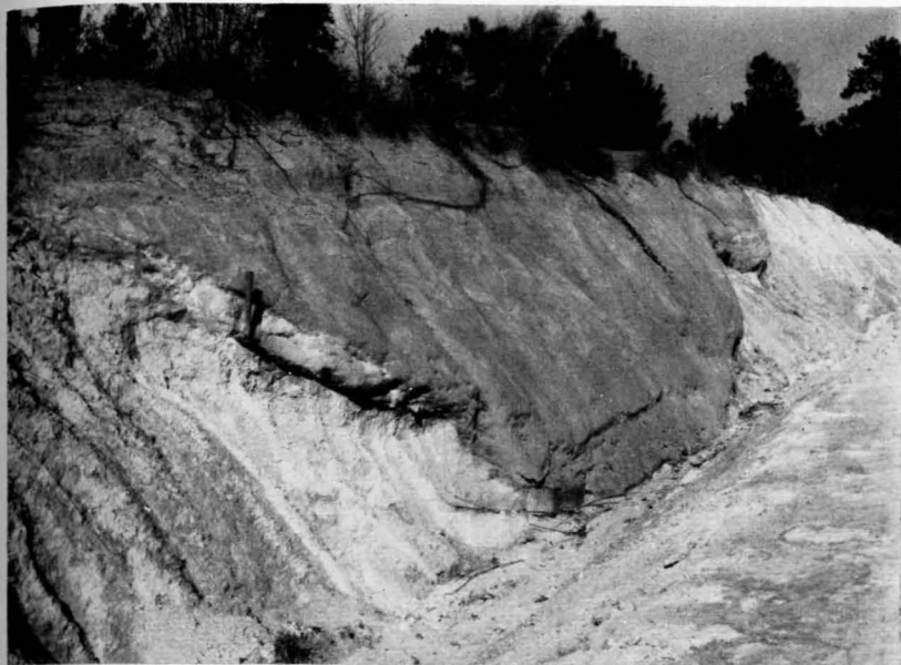
Figure 14. Exposure in road cut 1 mile east of Black Springs Church on Georgia Highway 22 (Baldwin County) showing pink coarse sand filling a channel in deeply weathered granite.
