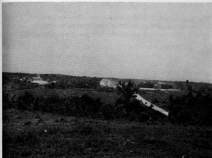
Figure 5. Talc mills at Chatsworth, viewed from the east; Georgia, Cohutta, and Southern Mills from left to right.
