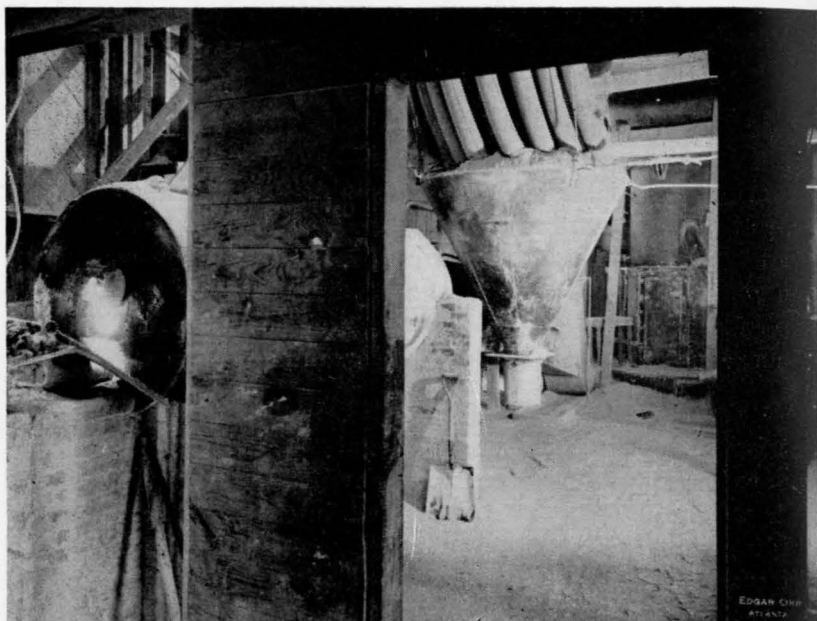
Figure 7. Flash dryer at Southern Mill used to dry damp talc; stocking collector used to trap air floated talc in right center, and Williams roll mill in background.
