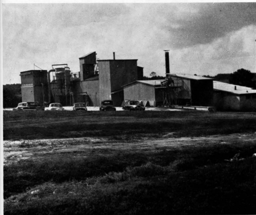
Figure 29.—A general view of the dry processing plant at the Funkhouser mine.
