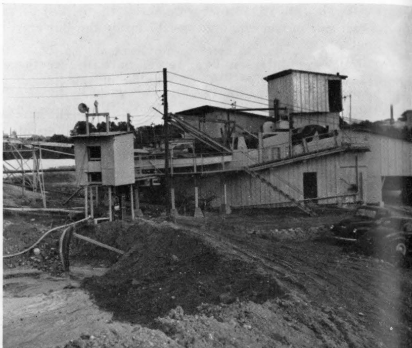
Figure 28.—A general view of the wet processing plant at the Funkhouser mine.
