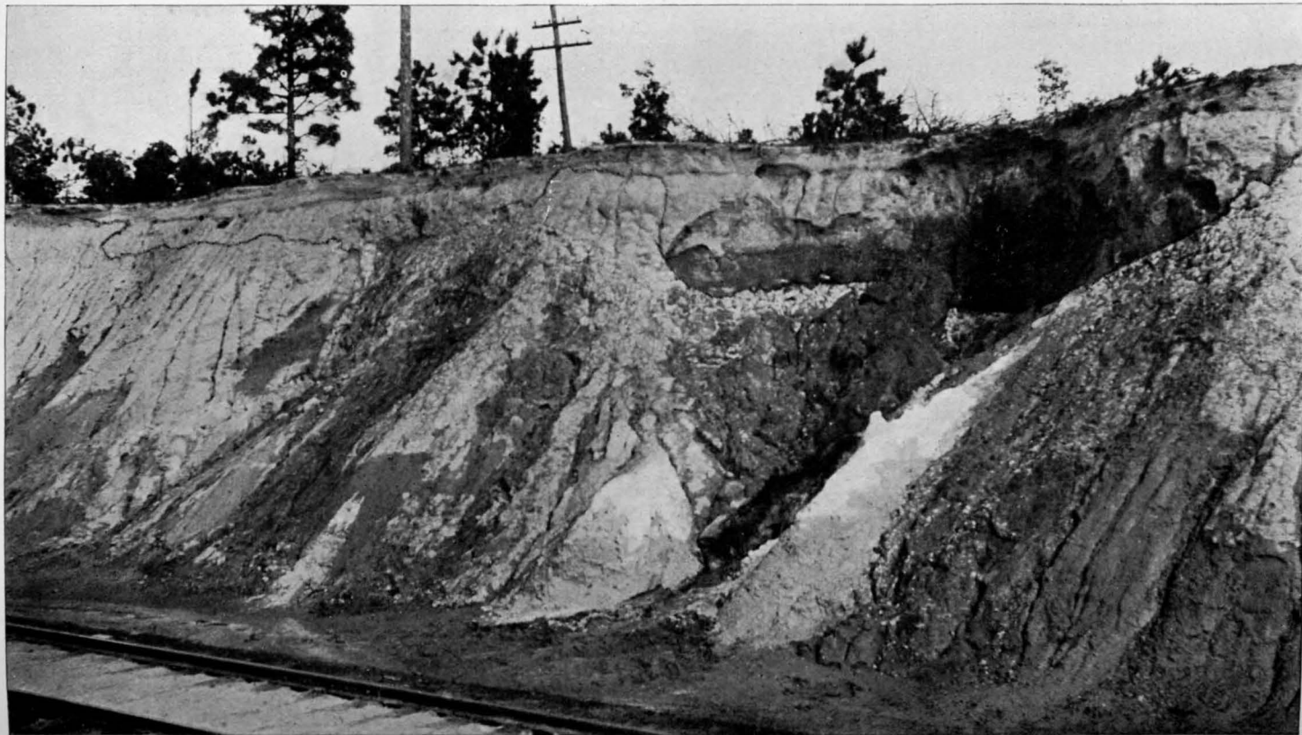
UNCONFORMITY BETWEEN SANDY CLAYS, IN A CUT ALONG THE GEORGIA RAILROAD, NEAR AUGUSTA, GEORGIA.
