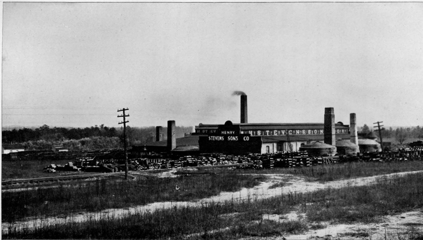
SEWER PIPE WORKS, MACON, GEORGIA.
