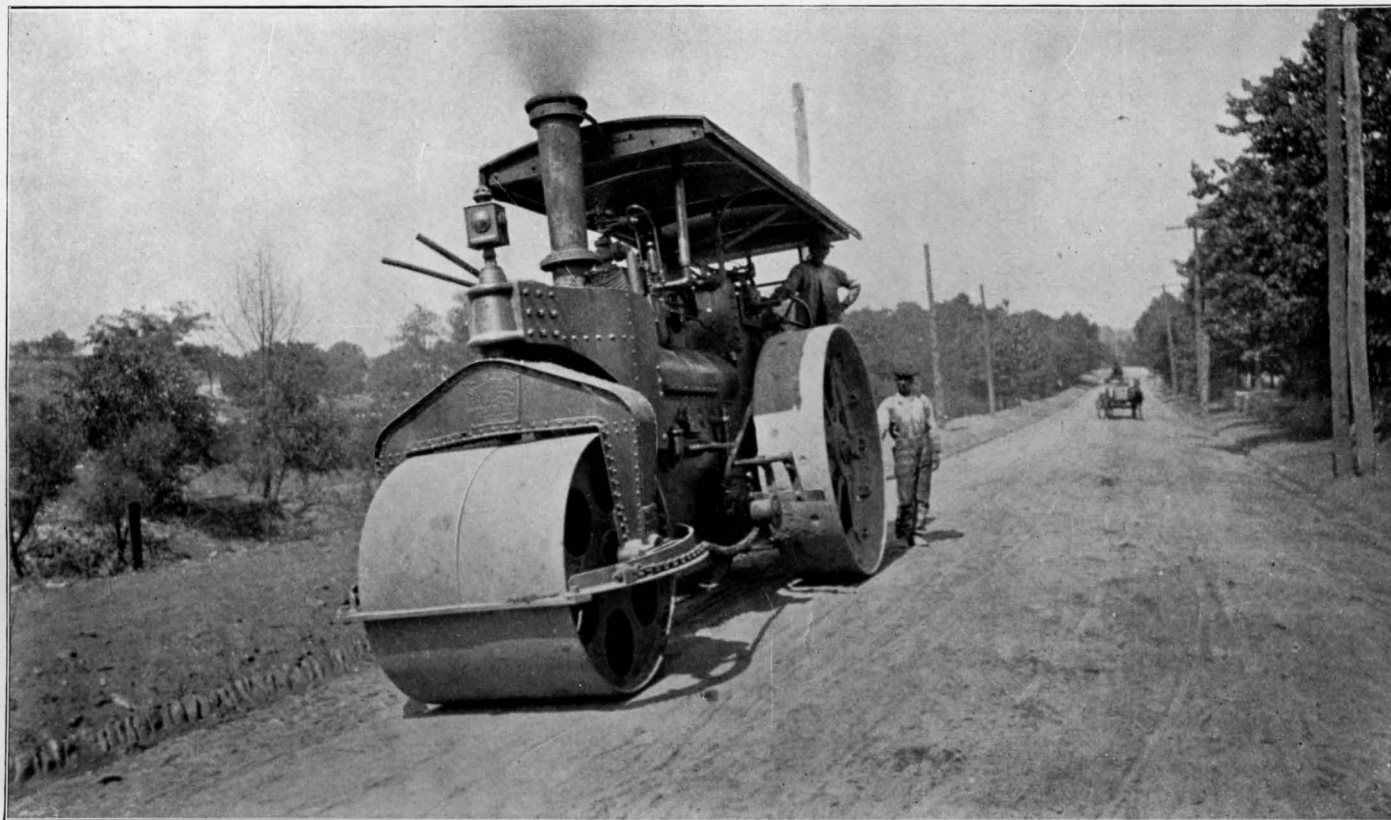
STEAM ROLLER AT WORK ON BATTLE HILL AVENUE, A SHORT DISTANCE BEYOND THE LIMITS OF ATLANTA.
