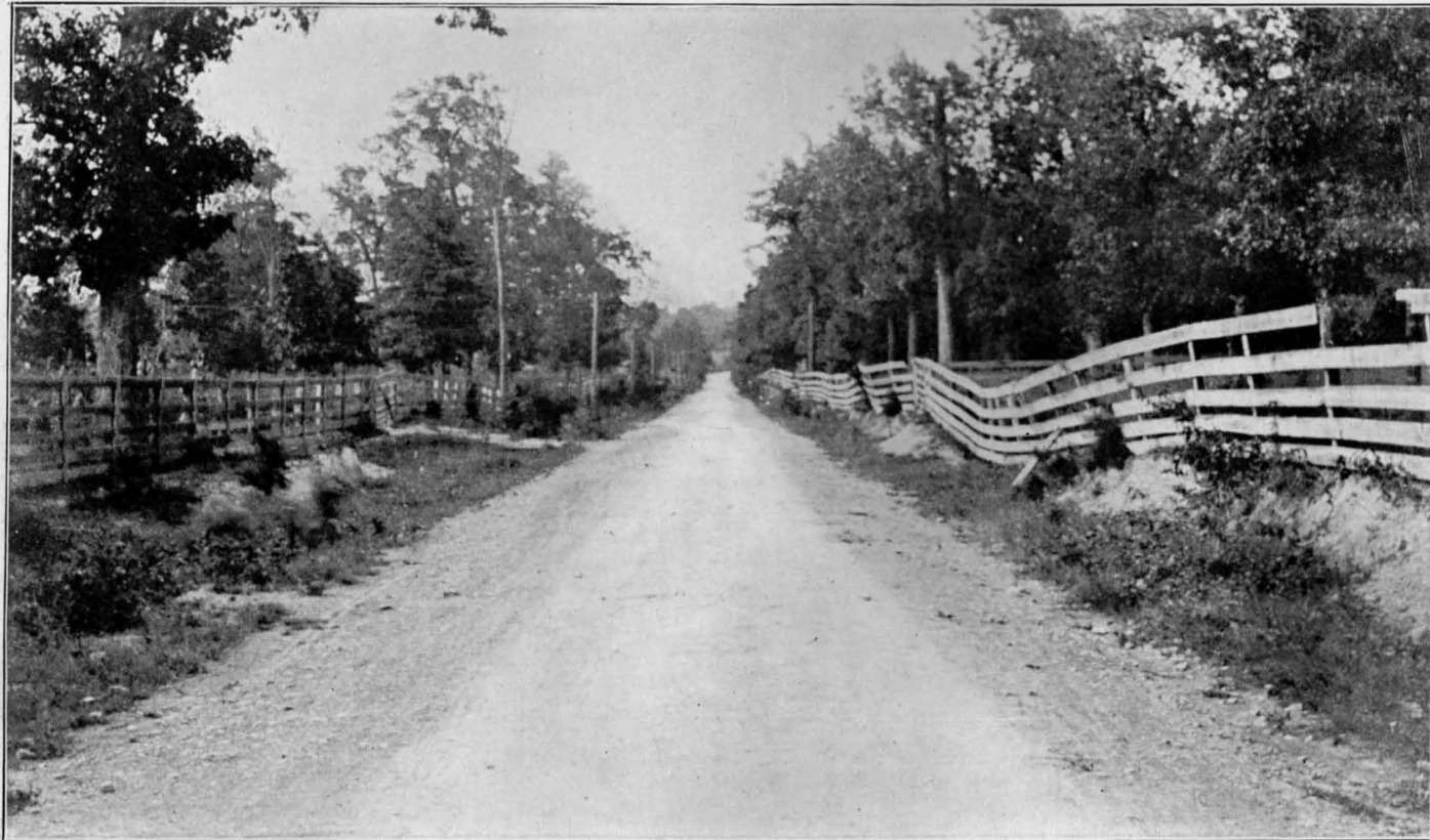
VIEW ON THE KINGSTON ROAD IN FLOYD COUNTY, 2 MILES FROM ROME, GEORGIA, SHOWING MACADAM CONSOLIDATED AFTER TRAVEL.
