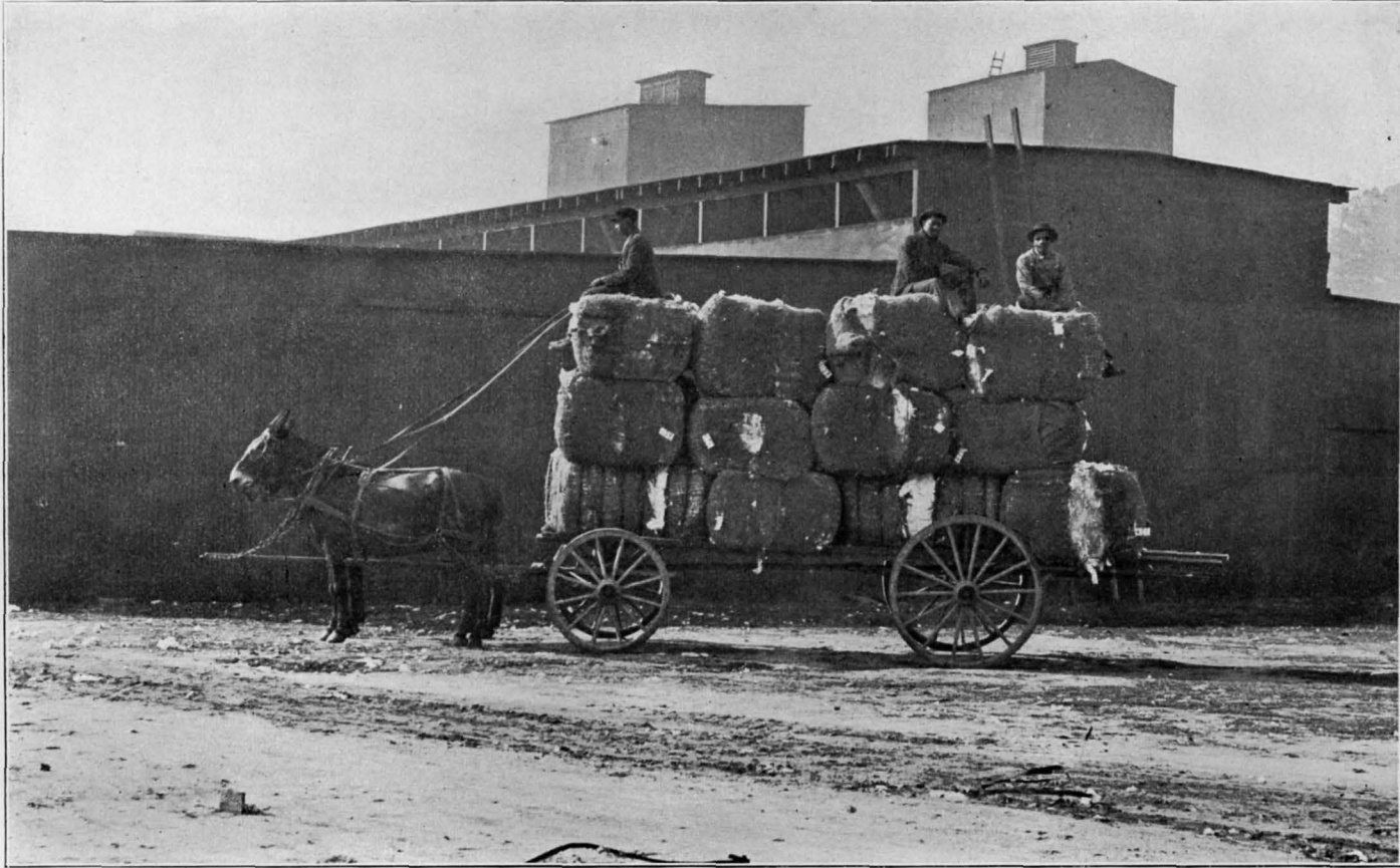
VIEW ON THE ROAD FROM AUGUSTA TO INMAN'S COMPRESS, RICHMOND COUNTY, GEORGIA, SHOWING A LOAD OF 12 BALES OF COTTON ON AN IMPROVED ROAD, INSTEAD OF 3 BALES, THE NORMAL LOAD ON AN UNIMPROVED ROAD.
