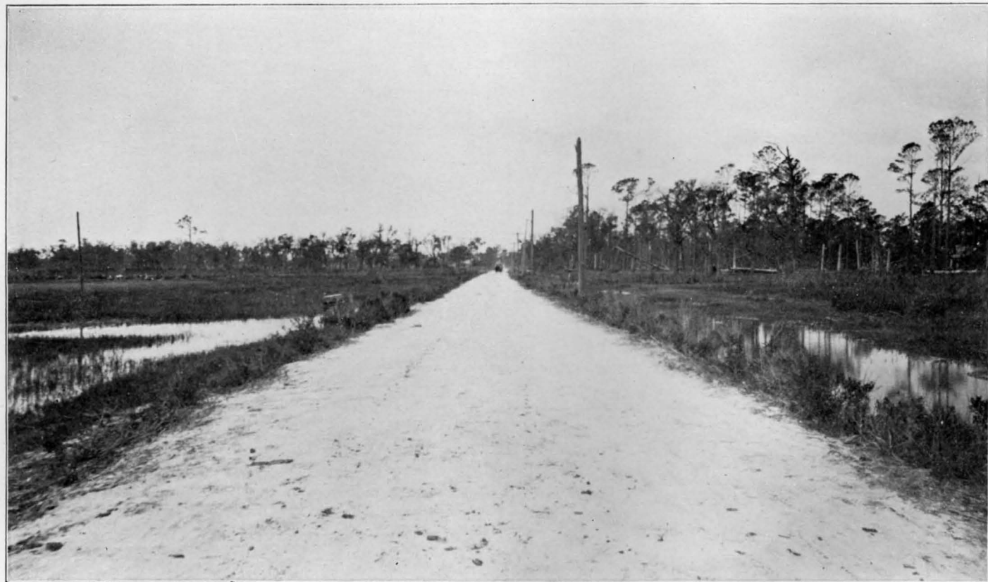
A CHATHAM COUNTY GRAVEL ROAD, NEAR SAVANNAH, GEORGIA.
