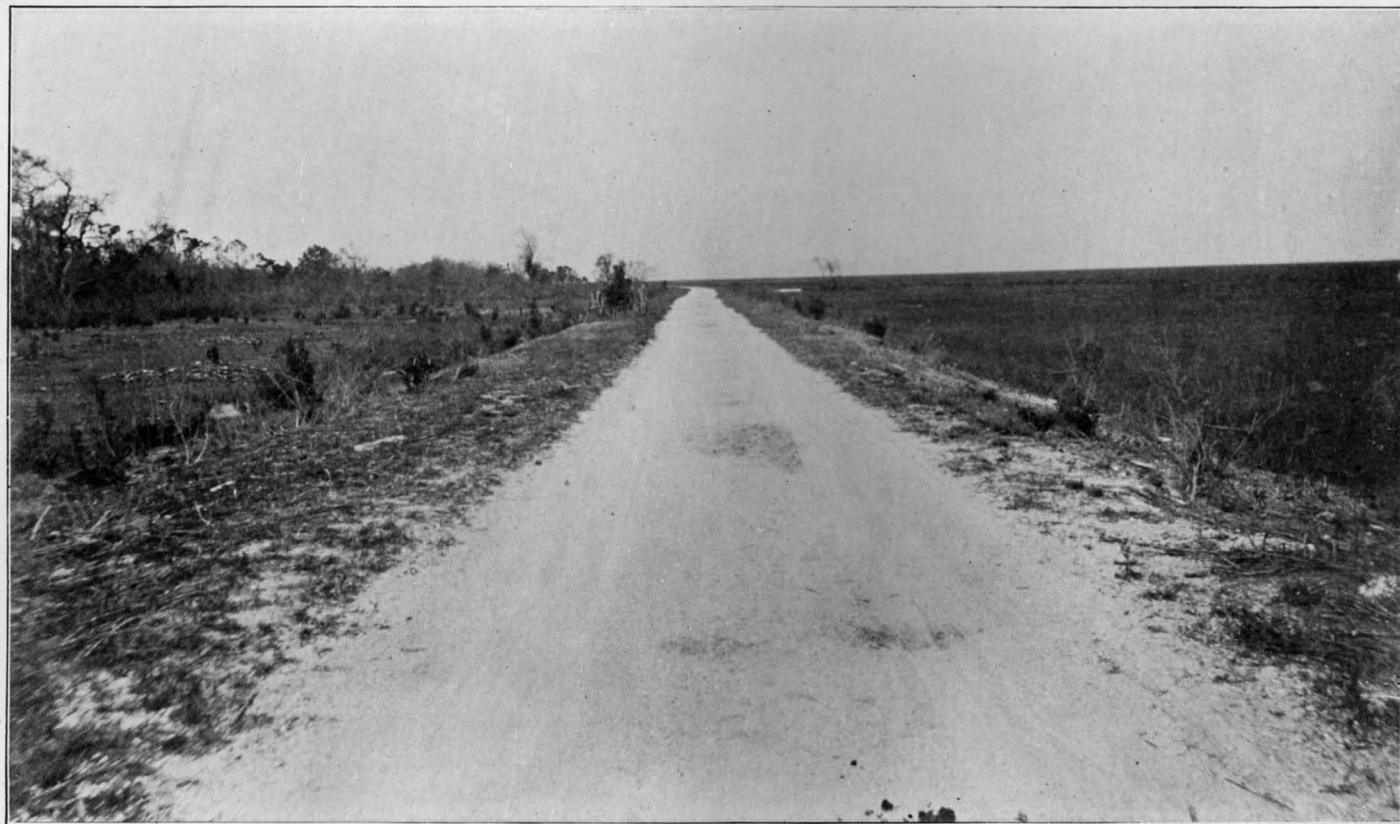
“ THE BOULEVARD ”—A SHELL ROAD ALONG A SALT MARSH NEAR BRUNSWICK, GEORGIA.
