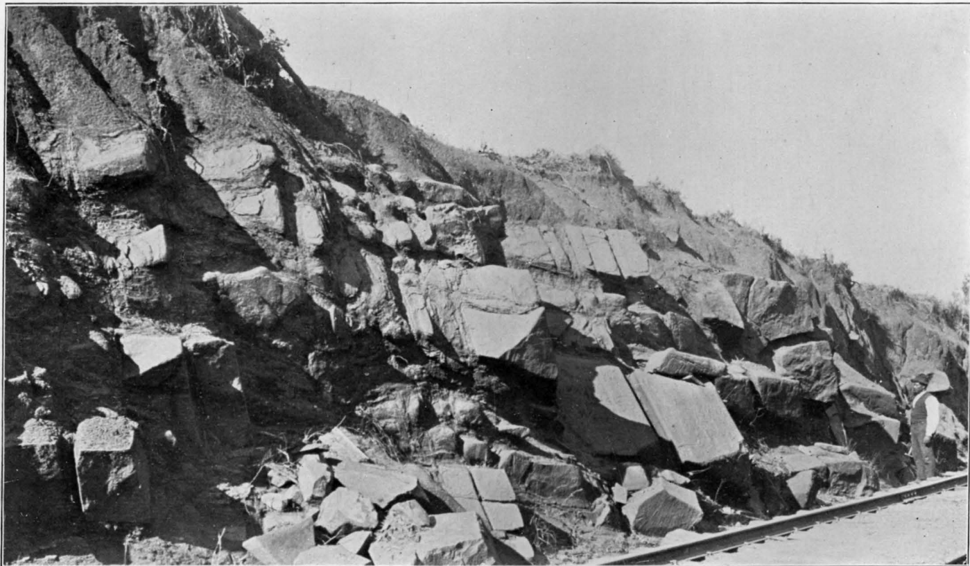
A TRAP DIKE IN A CUT ON THE MACON BRANCH, GEORGIA RAILROAD, NEAR ROBERTS STATION, GEORGIA.
