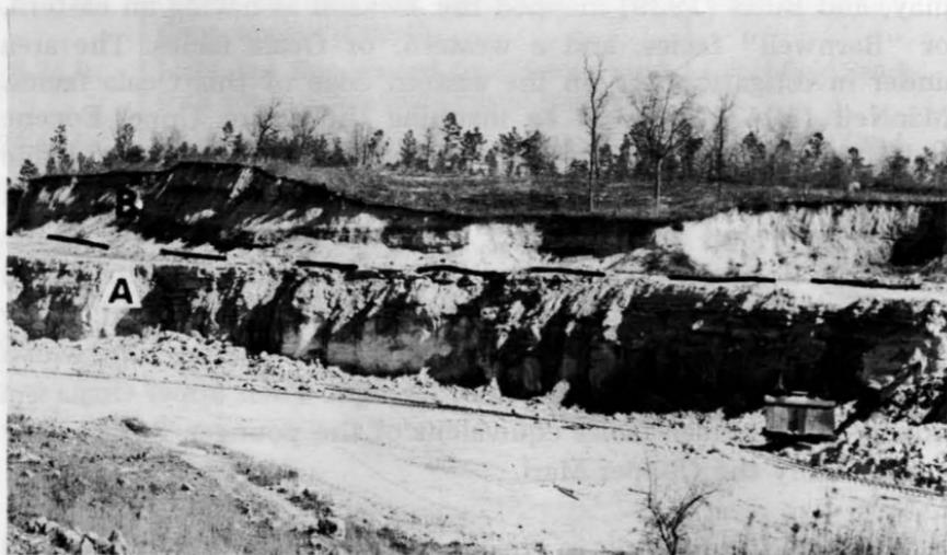
Figure 6. Ocala Limestone (A) and Twiggs Clay (B) at the old Clinchfield Penn-Dixie Cement Company east quarry, locality 10.
