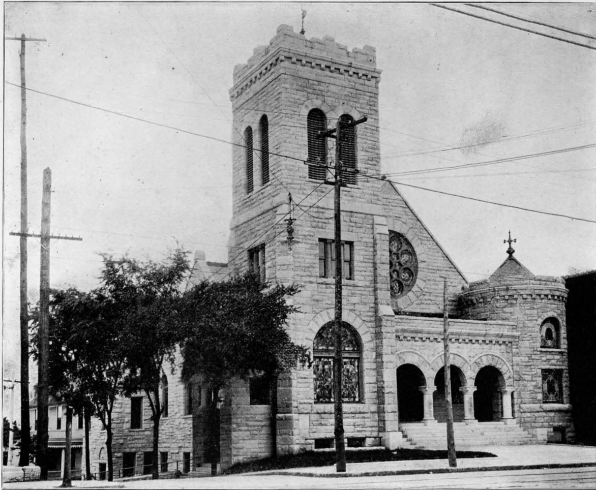
THE NORTH AVENUE PRESBYTERIAN CHURCH, ATLANTA, GEORGIA, BUILT OF STONE MOUNTAIN GRANITE.
