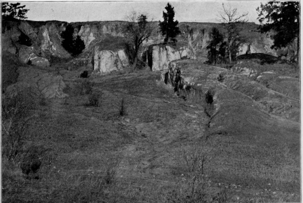
THE GREENVILLE GRANITE COMPANY'S QUARRY, NEAR GREENVILLE, MERIWETHER COUNTY, GEORGIA, AND THE ERODED SURFACE IN THE ACCOMPANYING RESIDUAL CLAY.
