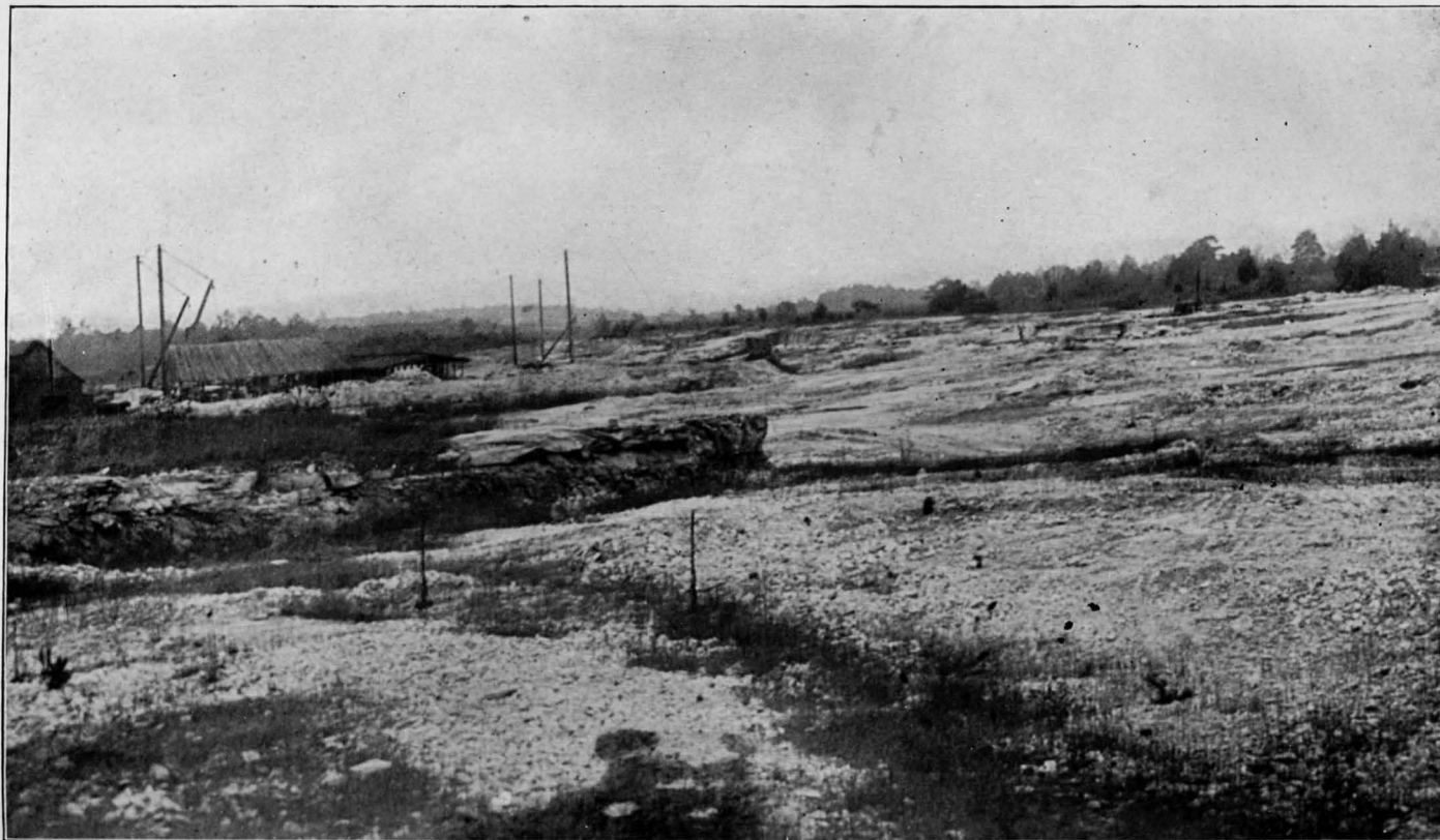
A GENERAL VIEW OF THE SOUTHERN GRANITE COMPANY'S QUARRY, NEAR LITHONIA, GEORGIA, ILLUSTRATING THE WORKING OF A FLAT-SURFACE OUTCROP OF GRANITE-GNEISS.
