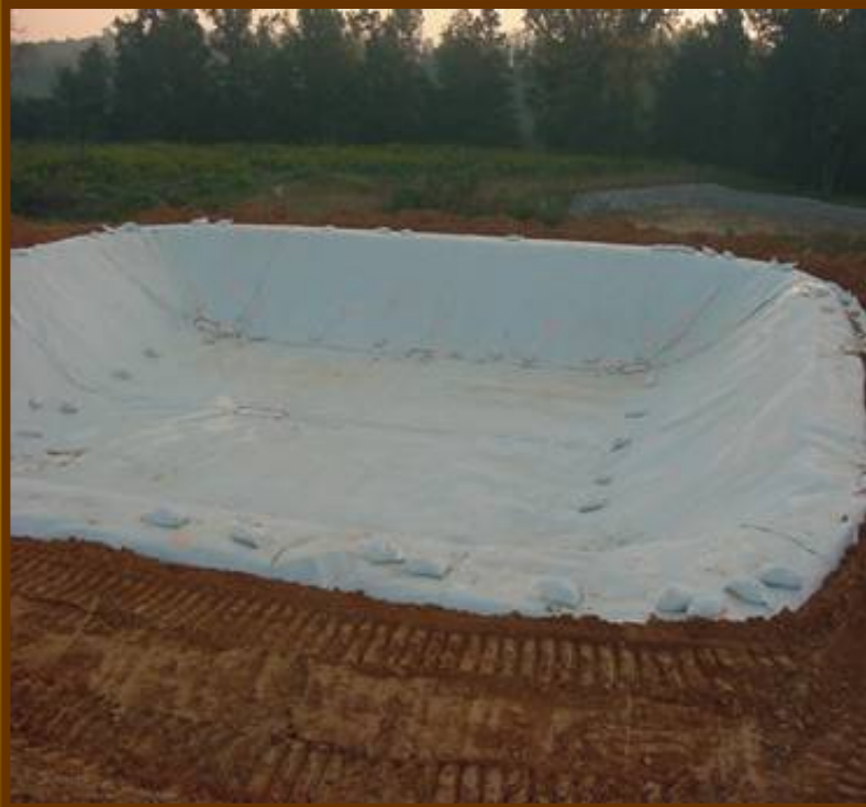
60 mil white liner installed for leachate pond
