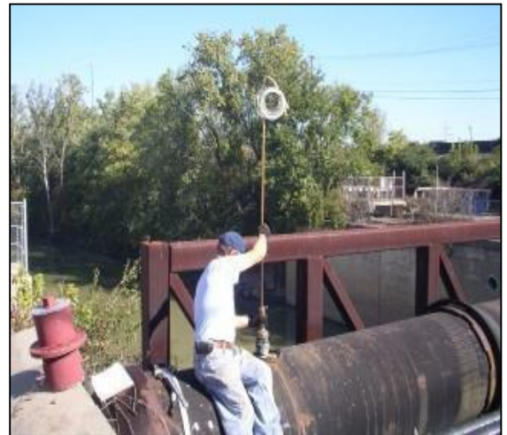
Figure 8 Pitot rod inserted into large pipeline
