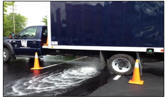
Figure 7 Meter testing via truck mounted apparatus
