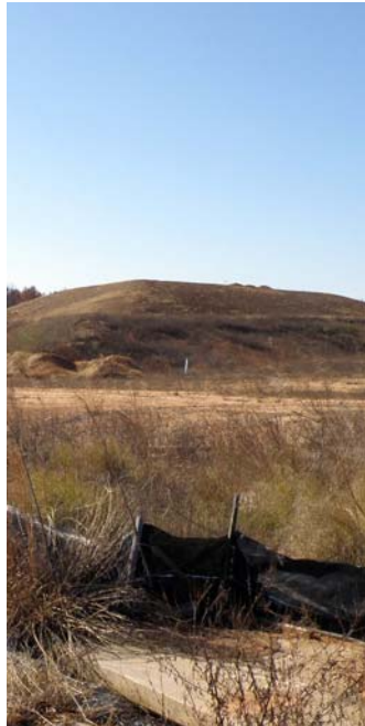
The Miller/Trammel Road Landfill in Forsyth County remains a risk for methane explosions.
