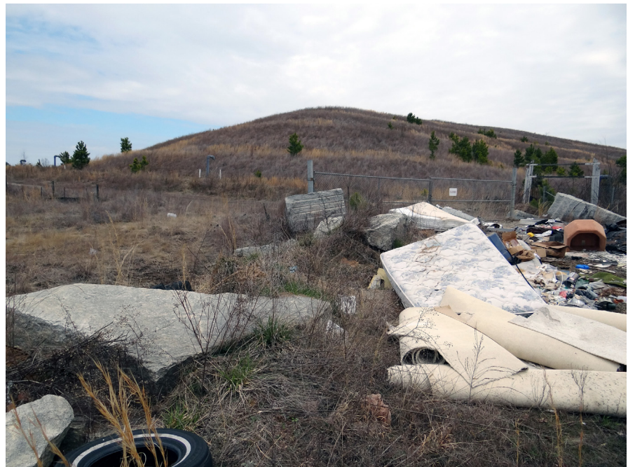
In the years since the landfill was closed, trees began to grow through the cap or cover damaging the cover system and uncontrolled access led to illegal dumping.
