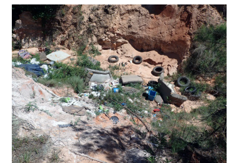
At the Fauconniere Buckeye Cellulose Industrial Landfill in Andersonville, the absence of an adequate final cover system led to trees and other vegetation becoming established and the formation of deep gullies due to erosion. Poor site access controls led to open dumping.
