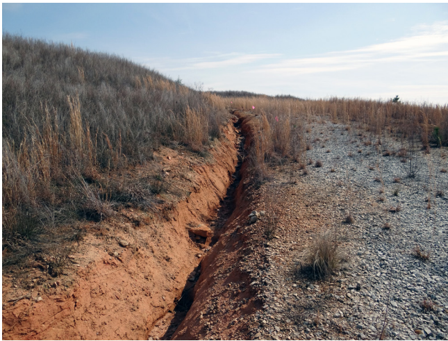
At the Scales Road Landfill in DeKalb County, the absence of an adequate final cover system led to the formation of gullies along some of the roads due to erosion (left). Contractors filled in the ditches as part of maintenance work at the site (right).
