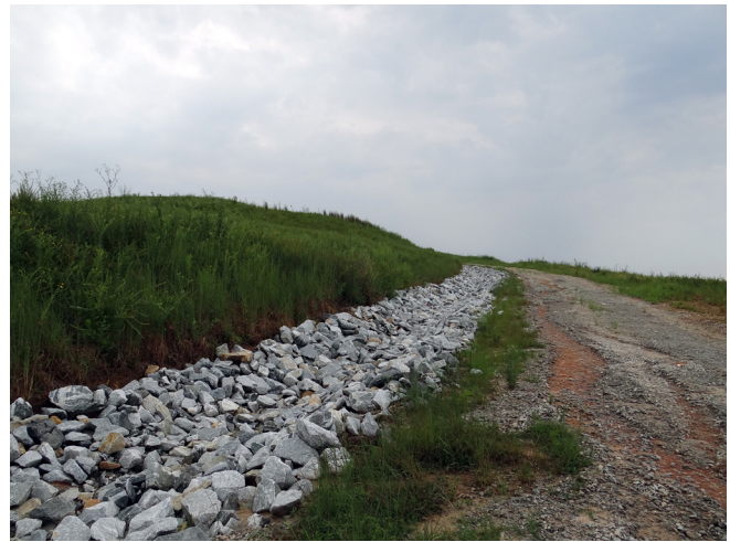
At the Scales Road Landfill in DeKalb County, the absence of an adequate final cover system led to the formation of gullies along some of the roads due to erosion (left). Contractors filled in the ditches as part of maintenance work at the site (right).
