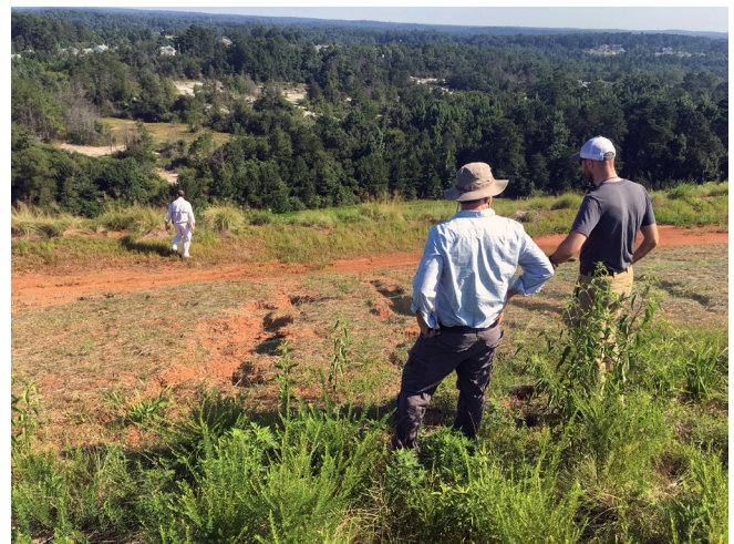
Maintenance activities at Scales Road also include maintaining the integrity of the landfill cap to ensure proper vegetation is established. In the photo above, EPD staff perform an inspection of the site along with a representative from the contractor company.
