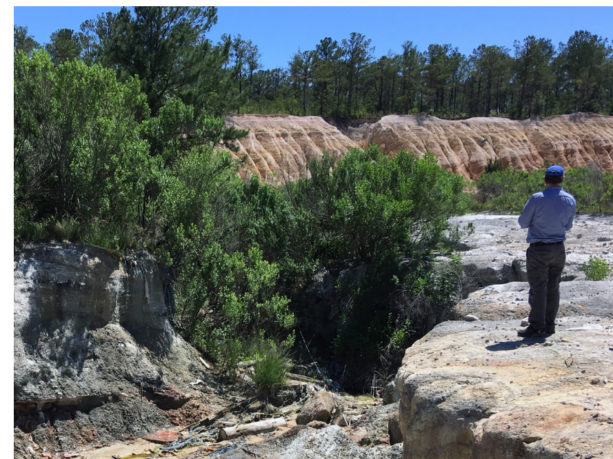
At the Fauconniere Buckeye Cellulose Industrial Landfill in Andersonville, the absence of an adequate final cover system led to trees and other vegetation becoming established and the formation of deep gullies due to erosion. Poor site access controls led to open dumping.
