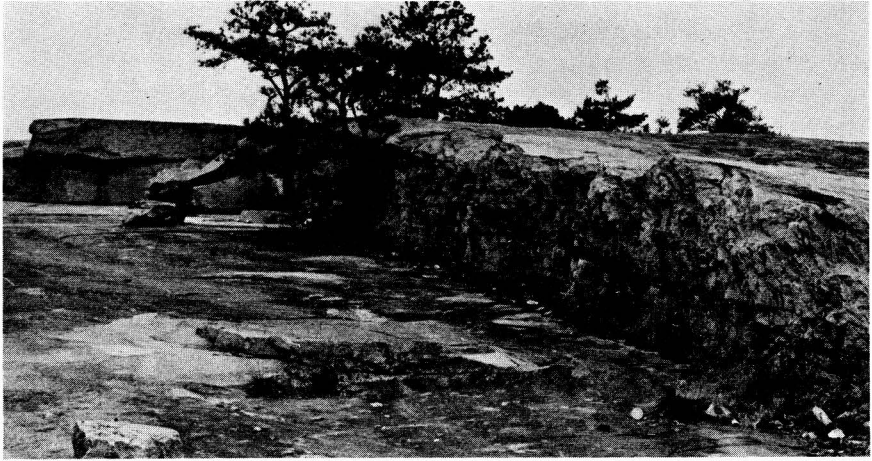
Figure 16. Quarrying—Opening the ends
