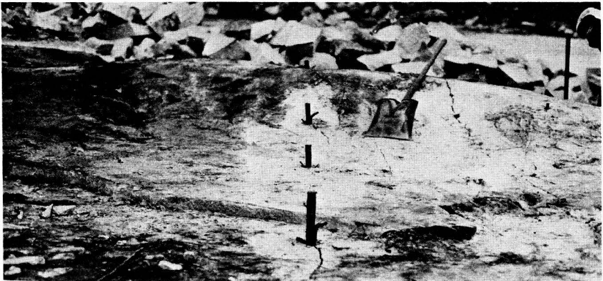
Figure 17. Quarrying—Opening of the break.
