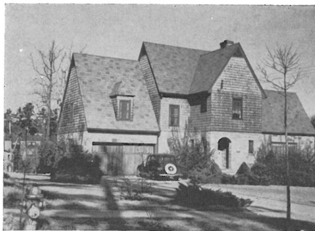
House in seam or strata face ashlar finished off with wood shingles of similar color.
