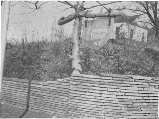
A strip rubble wall. The Street Marker also is of slate.
