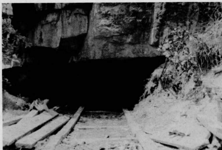
Figure 14. Coal Opening on Lot 55, District 19. Thirty-three inches of coal may be seen to left. This is typical of the individual coal mines operating in the Sand Mountain area.
