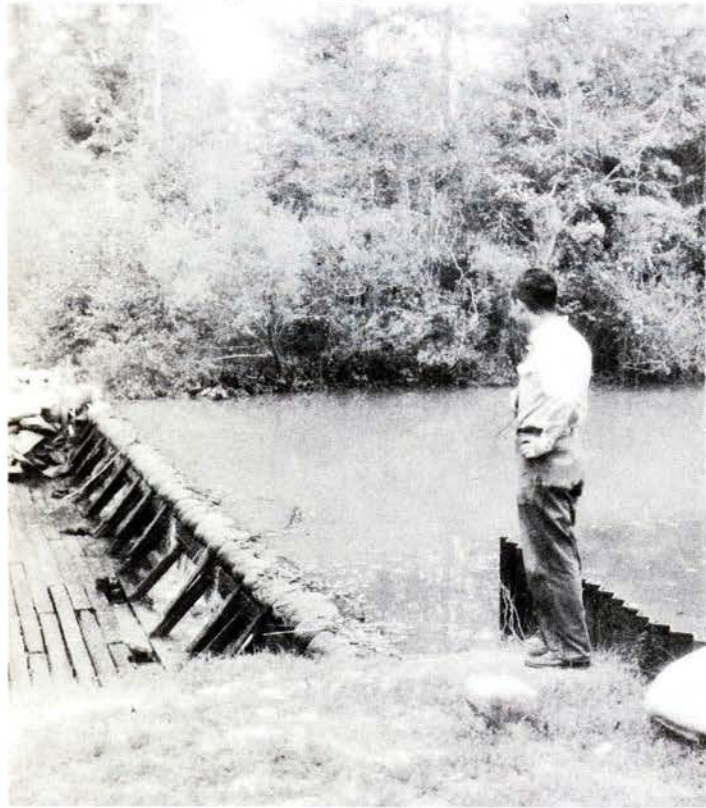
Fig. 2. Sandbagged water supply dam on Flint River near Griffin. At times during the drought the entire flow of the river at this point was pumped into the City water mains.
