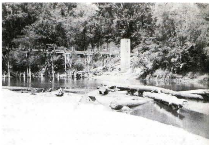
Fig. 10. Gaging station on the Ogeechee River at Scarborough, Ga., during the 1954 drought. The concrete tower encloses a well that is connected to the river by pipes. The upper part of the tower is a shelter for the recording instruments.
