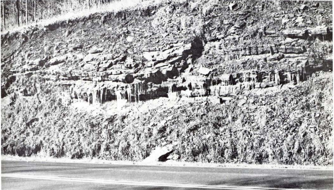
Figure 9. Icicles form where ground water leaks out of the Red Mountain Formation along steeply inclined bedding plane openings.
